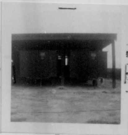
Trailers under a Shed
