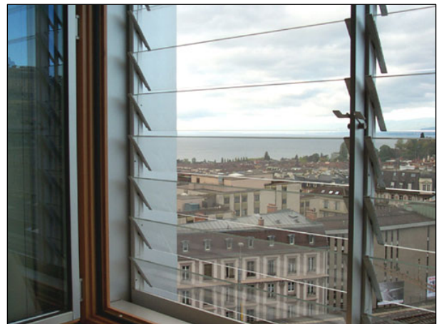
Figure A-86 Moveable glass louvers interior
