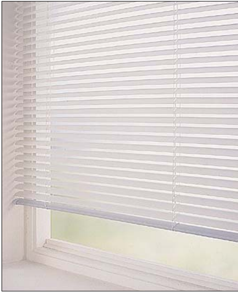
Figure 4-11 Existing shading device system – vinyl light grey blinds
