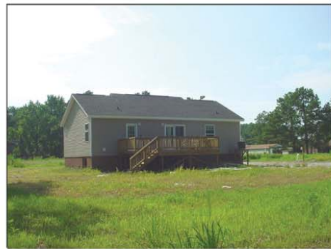
NEW CONSTRUCTION ADJACENT TO THE SOUTH WEST BOUNDARY
