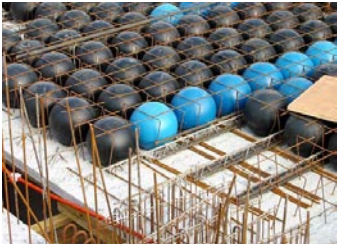
Bubble deck under construction
