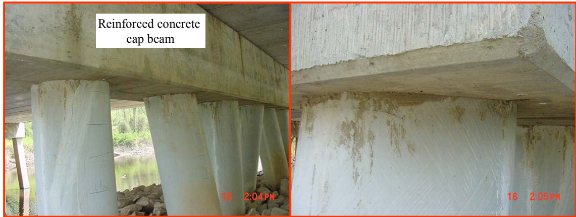
Figure 5.27 Pier no. 2 including the composite piles and reinforced concrete cap beam
