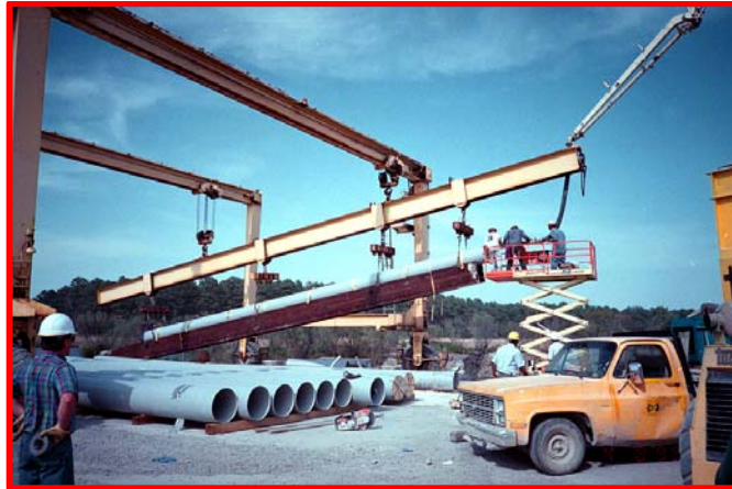
(a) Pumping concrete into the upper end
