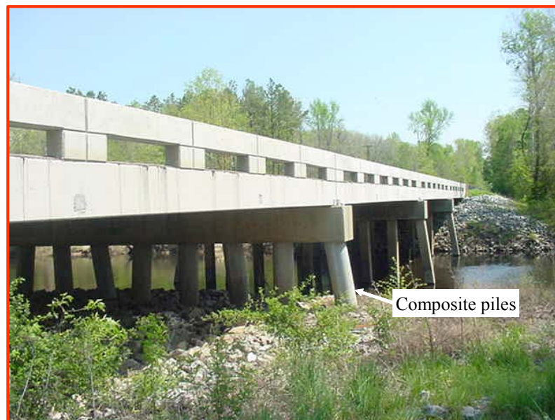
Figure 5.28 The new Route 40 Bridge over the Nottoway River in Virginia
