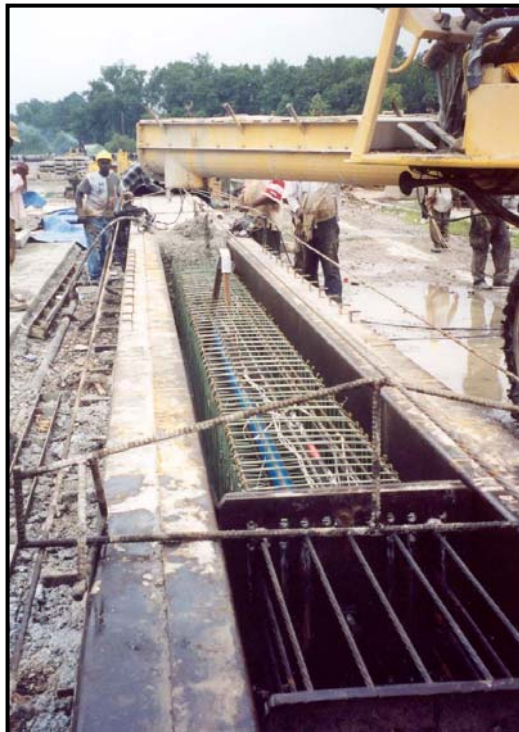
Figure 5.9 Fabrication of prestressed concrete pile
