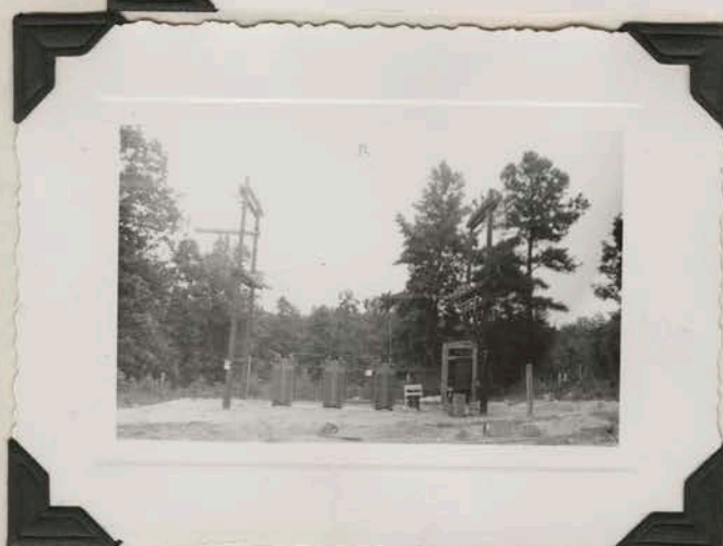
Farmers Rural Utilities substation under construction near Bowling Green, Caroline County. This station will supply approximately 400 miles of distribution lines with current.
