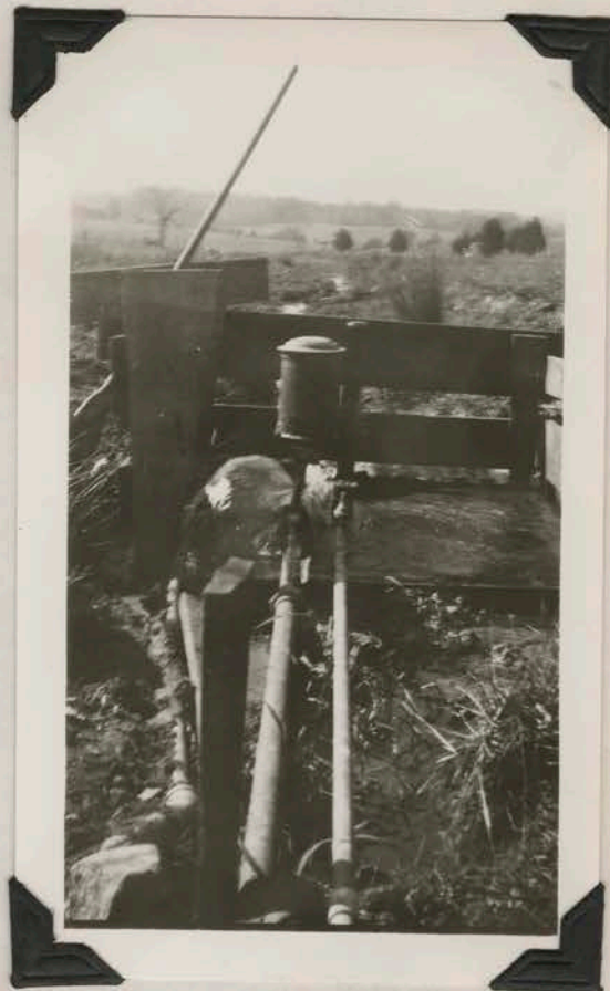
A hydraulic ram and overhead tank -- probably one of the most used and certainly one of the cheapest methods of home water supply.
