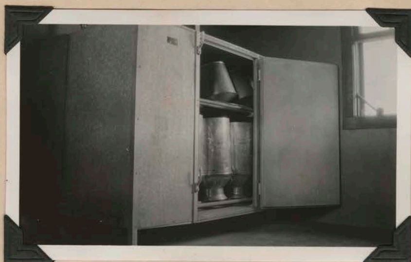
Dairy sterilizing cabinet. Required on Washington market.
