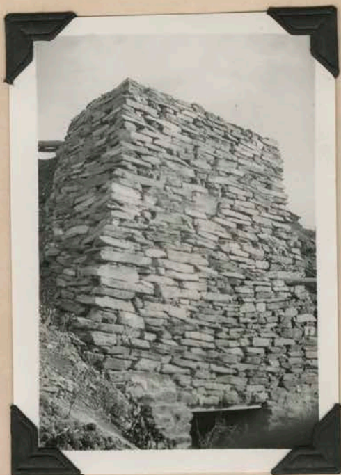
Two views of a permanent type lime kiln in Smyth County. Cost, including compressor for drilling rock, $750.00. Size 6 ft. in diameter, 25 feet high. Produces 3½ tons per day. This kiln has been burning continuously since January 1936.
