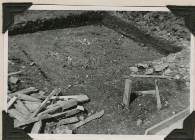
Excavation for a permanent electric hot bed.
