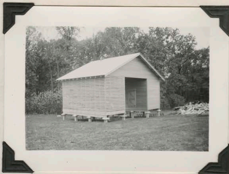
Center drive corn crib in Orange County. Plan J-1.12
