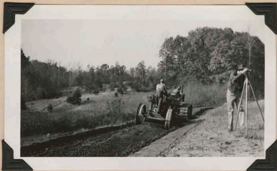
Laying out and building terraces in Pittsylvania County
