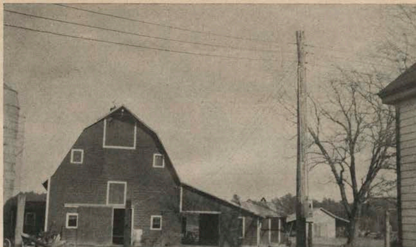
Meter pole and distribution center on a dairy barn in Virginia. There are many advantages and economies in this type of meter installation.
