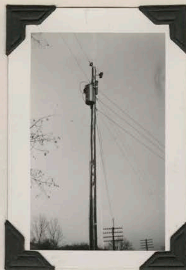
Secondary wires leaving 6900 volt transformer to serve three customers.
