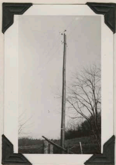
Branch line leaving 6900 volt single phase line.
