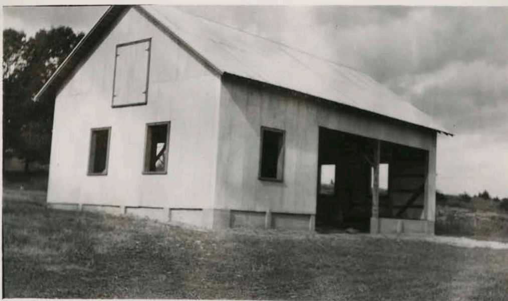
Two views of the two-story community machine shop built by the Ottoman Farmers' Cooperative, Inc. in Lancaster County. The building houses a forge, wood working shop, metal working machinery and a seed cleaning mill.
