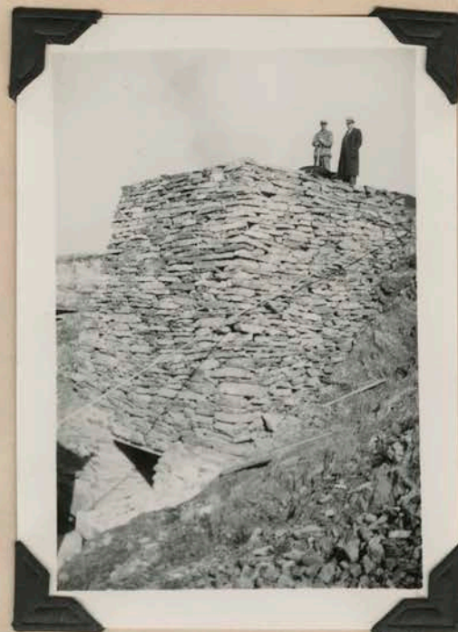
Two views of a permanent type lime kiln in Smyth County. Cost, including compressor for drilling rock, $750.00. Size 6 ft. in diameter, 25 feet high. Produces 3½ tons per day. This kiln has been burning continuously since January 1936.
