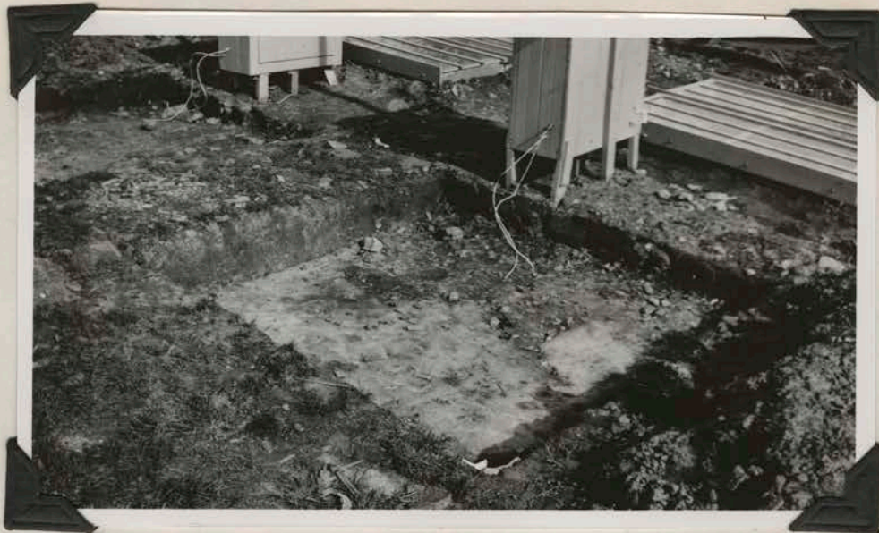
Electric hotbeds under construction. Two beds have sashes in place. Note houses for instruments.
