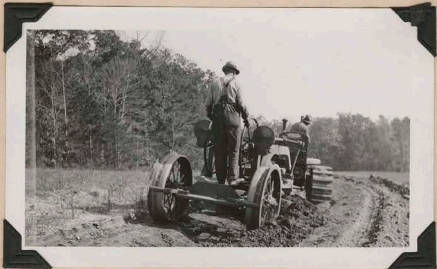
Cutting terrace channel - Pittsylvania County
