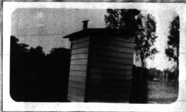
New sanitary toilet on the farm of William Jones Carson, #2.
