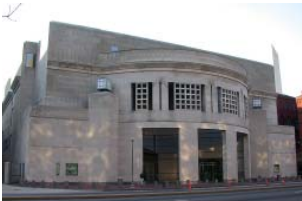
Figure A-1. 14th Street entrance.
