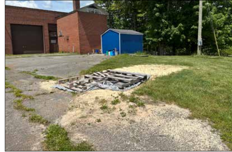
14: The sand jump pit, implemented for track and field practice, erodes into the adjacent parking lot during rain events and becomes hazardous for athletes.
