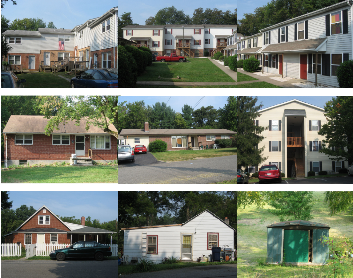
Existing buildings on Tee Street
