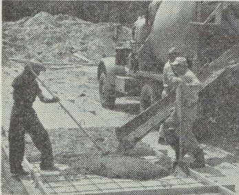
Wall panels are cast on floor
