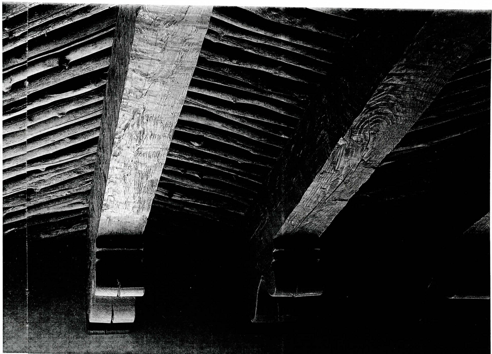
A family of means could have vigas hand adzed to form square beams. These beams, with carved corbels at each end,
