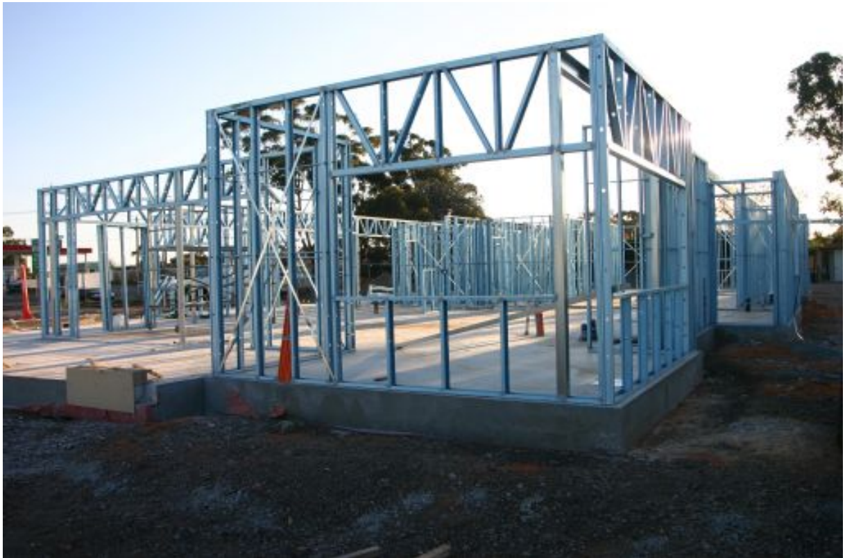
Picture 1.1.1. – A typical cold-formed steel application
