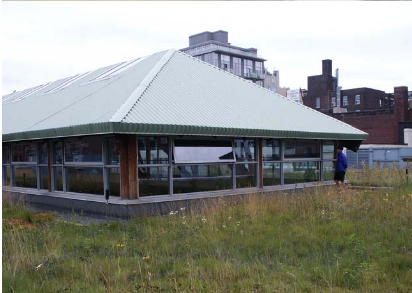
The green roof surrounds the roof monitor.
