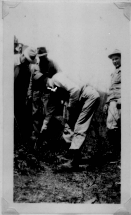
Mr. Waller, Agricultural Engineer, V.P.I., places dynamite for a ditching demonstration.
