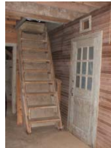
Stairs to the loft area
