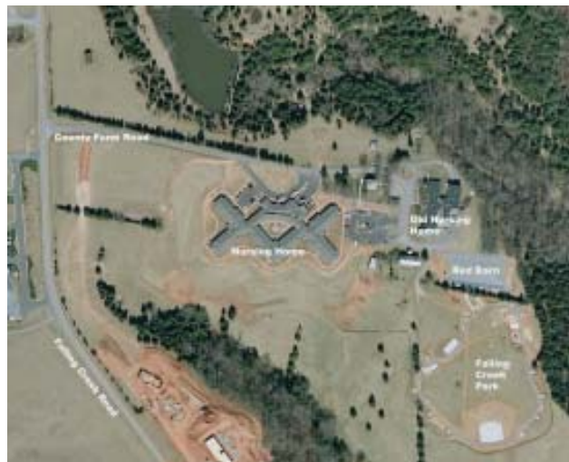
Aerial view of the County Property
