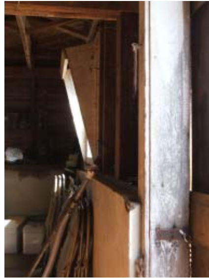
Door frame and studs on concrete wall
