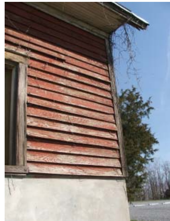
Siding on the southern side of the barn
