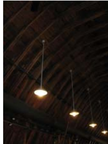
Homestead loft ceiling
