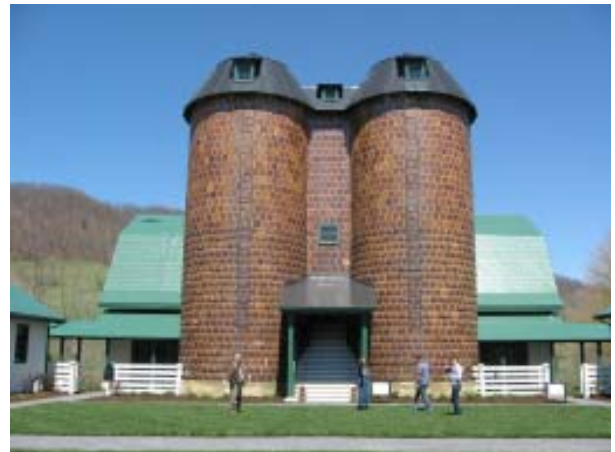
The renovated barn with tile silos
