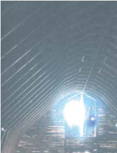
Red Barn loft ceiling
