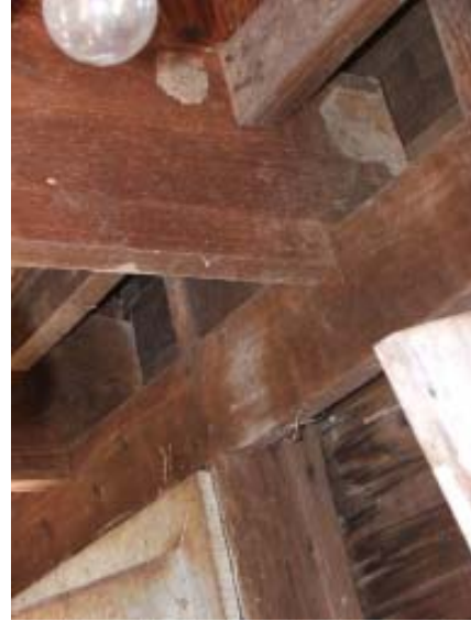
Joists and beams
