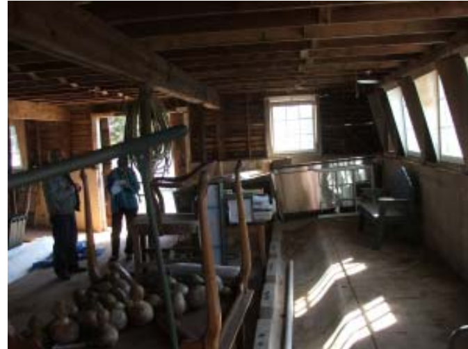
First floor feedway and windows
