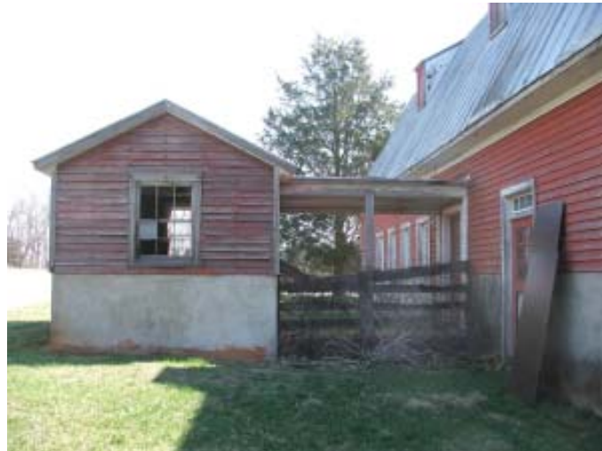
Western side of adjacent building; perhaps formerly a milk storage room
