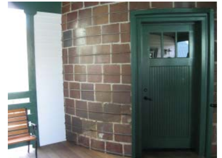
Door in tile silo
