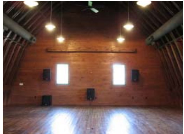
Homestead Dairy Barn loft center view. A large screen is hidden within the horizontal piece of wood. Rather than hurt the architectural integrity of the building by formally hiding ductwork, it was unobtrusively incorporated.
