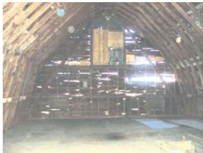
Loft western wall
