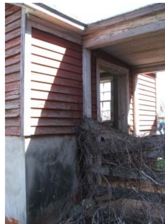
Southern side of adjacent building
