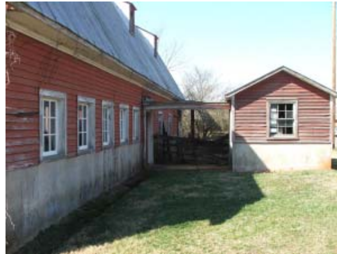
Eastern side of the adjacent building
