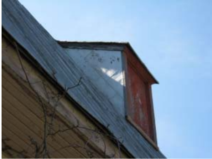
Dormer on roof
