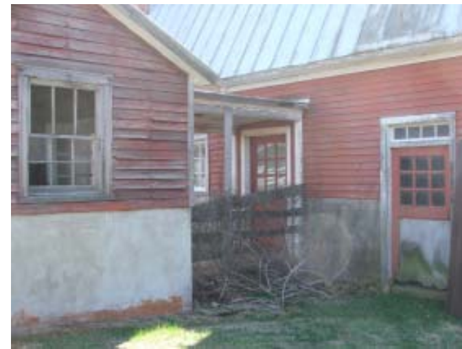
Northwest side of the Red Barn with adjacent building
