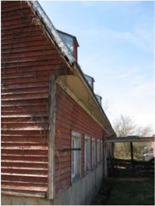
Dormers on the roof on northern side of barn
