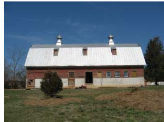
Southern view of the Red Barn
