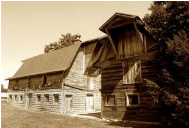
Barns at Rose Hill before renovations
