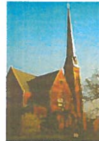
The Old West End Historic District in Danville contains one of Virginia's most concentrated collections of Victorian and 1900s residences. The First Baptist Church sits on Main Street. Listed on the registers in 1973
