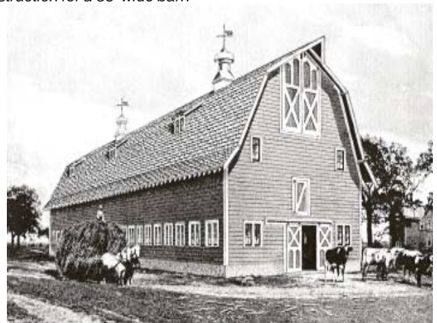
This image depicts some similarities to the Red Barn including the hay doors and how they open and the sliding main doors. However the roofline differs.
