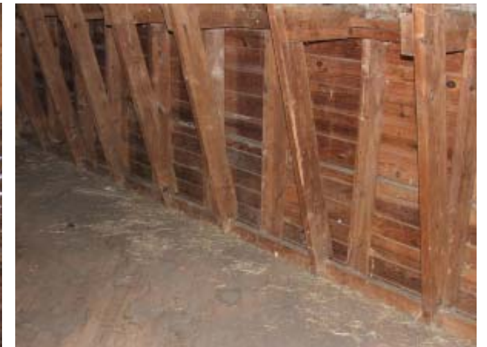
Construction detail close up
