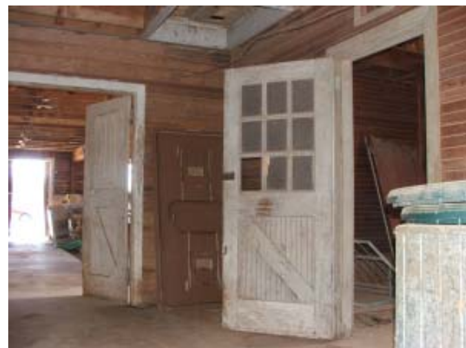
Middle section looking southeast
