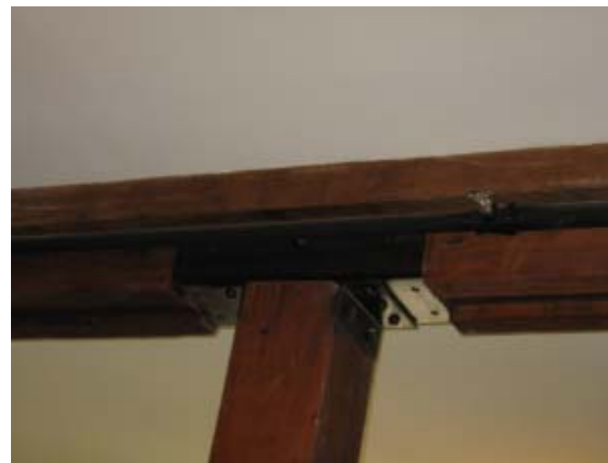
Interior construction detail
