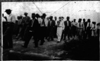
Working Along to East Demolition
