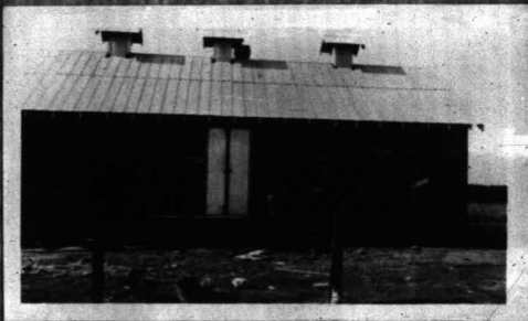
Water Wash House - 2,000 Barrel Capacity
