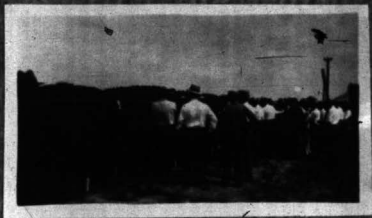
Men working High Water at East Avenue Demolition
