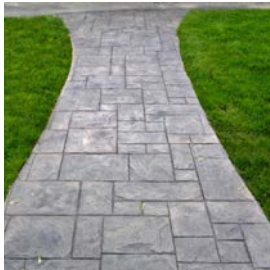
Stamped concrete sidewalks create visual interest at a lower cost.
