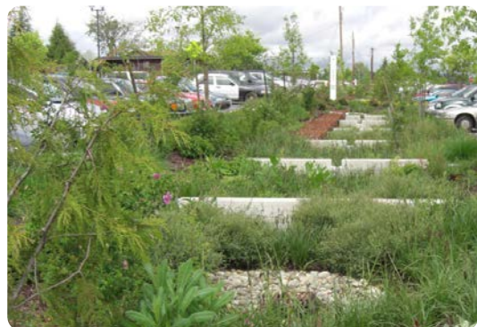
Using permanent and non-permanent structures to create an effective rain garden.
