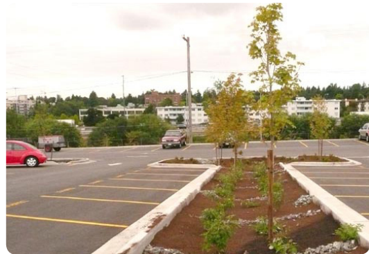
Rain gardens in parking lot islands can help to slow infiltration and hold water.
