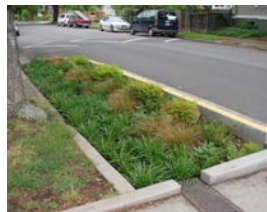
Bio-retention along a street corridor.
