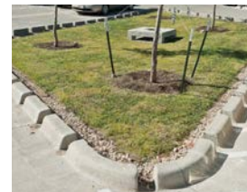
Bio-retention island within a parking lot.
