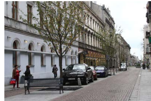
This woonerf shows the lack of curbs, creating more of a plaza than a road.
