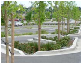
Bio-retention in a parking lot.
