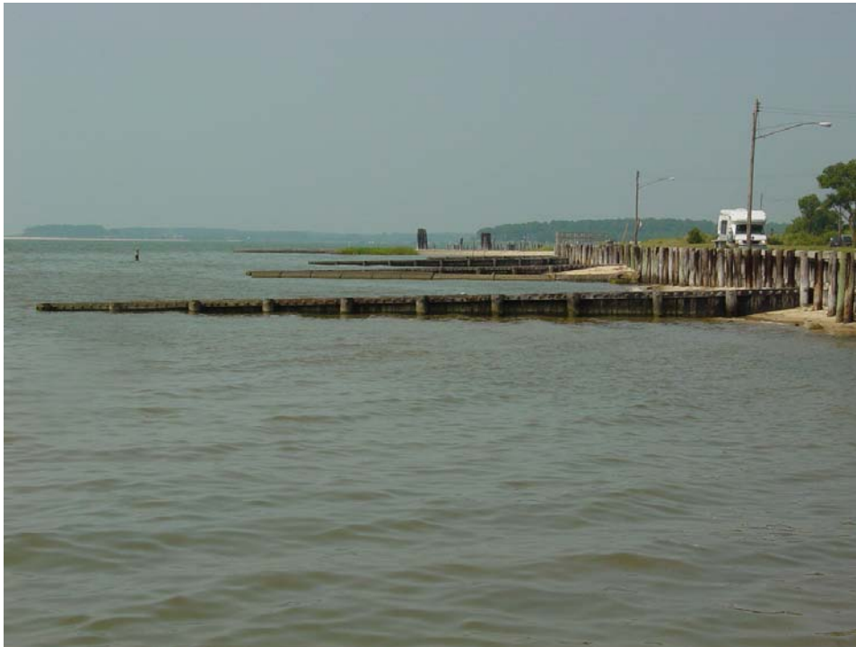
Picture 16 – Numerous SDs and groins visible on the northern end of Cape Charles beach. Numerous birds were observed on these structures, but are not visible in the picture.
