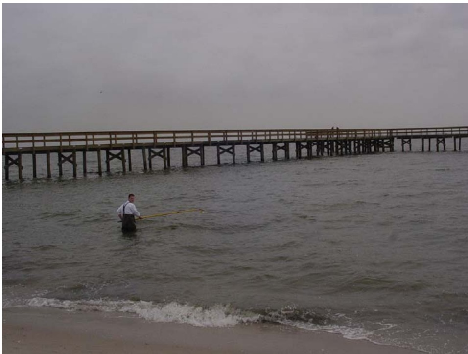
Picture 6 – Collecting samples at King-Lincoln A in 2005 with rebuilt pier visible in the background.
