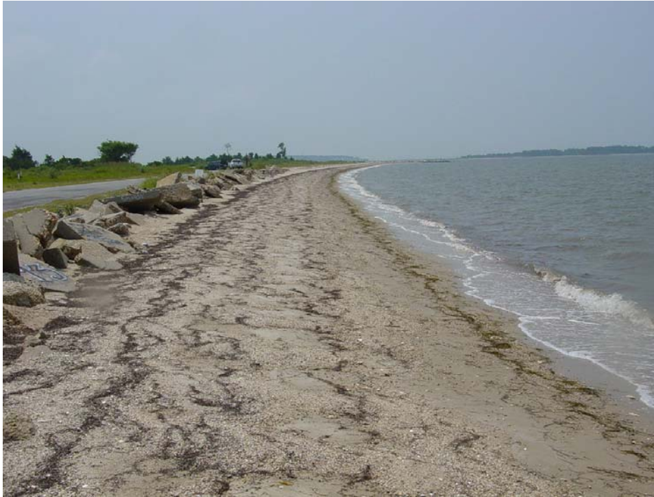
Picture 15 – Looking southward down the length of Guard Shore beach
