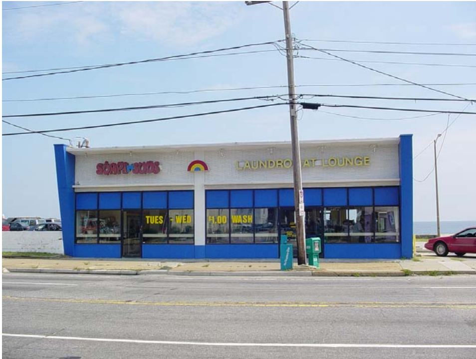
Picture 10 – Laundry mat immediately behind Norfolk SD-E and SD-W just off the beach. This facility is suspected of being illegally connected to SD-E and the source of extremely high fluorometric readings and visible soap bubbles in collected samples.
