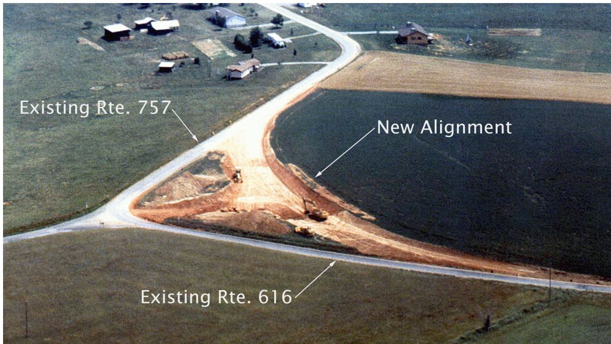
Figure 3.1 Original road and new alignment section
