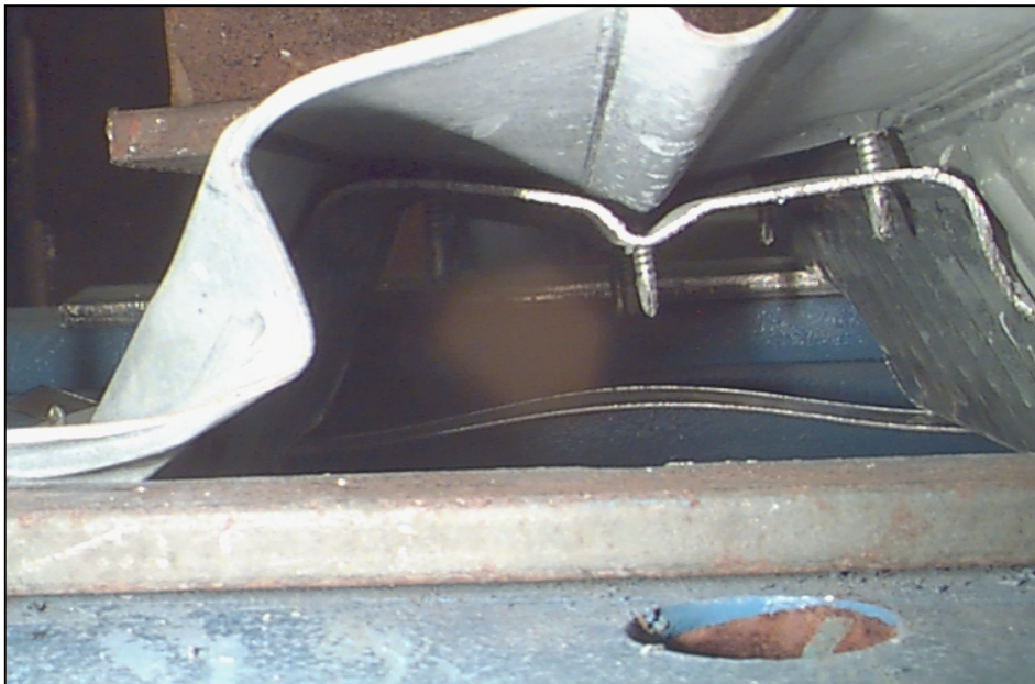
Figure 3.15 Crippled 3VLI-Deck
