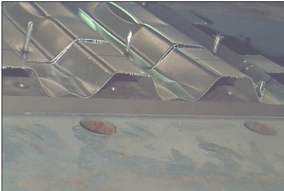
Figure 3.11 Crippled HD-Deck
