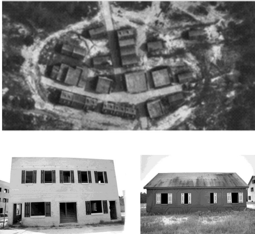
Figure 6.1: Overhead satellite image of the McKenna MOUT site at Fort Benning and individual building details (below) [94].
