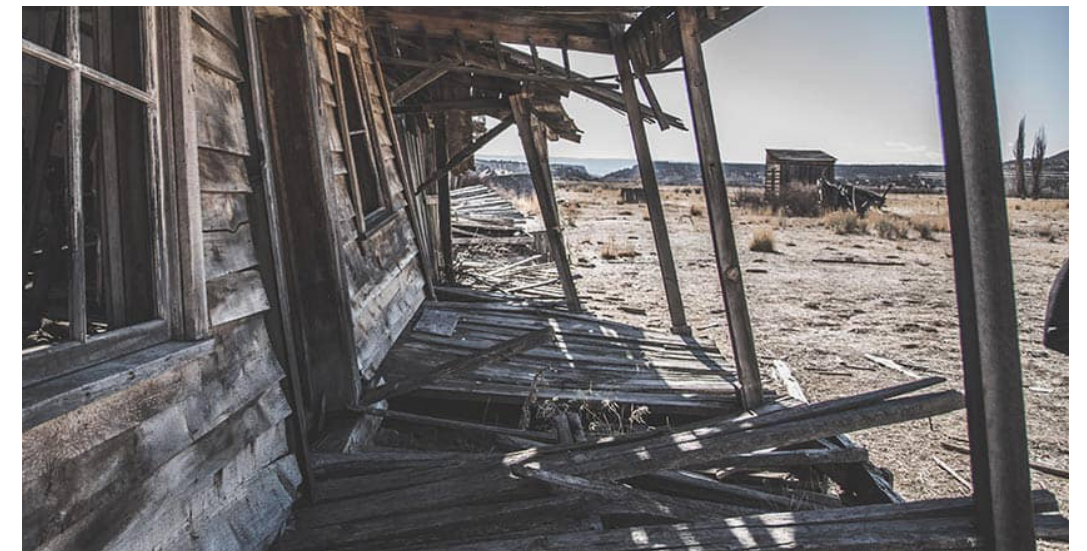
Figure 4: Wrong material A house in France built in 1912.
