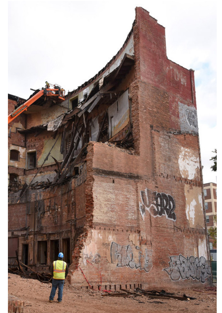
Figure 50: The Mayfair Theater After Partial Demolition in 2016.
