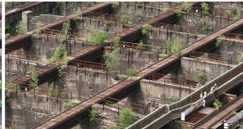
Figure 19: The Ore Bunker Gallery, Passages
