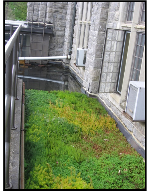
A "green roof" demonstration on Virginia Tech's Seitz Hall, April 2010. Green roofs are intended to reduce rooftop stormwater runoff.
