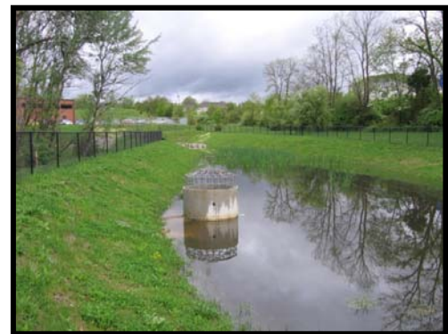
A stormwater-detention pond at the Moog Components Group facility in Blacksburg, Va., April 2010.
