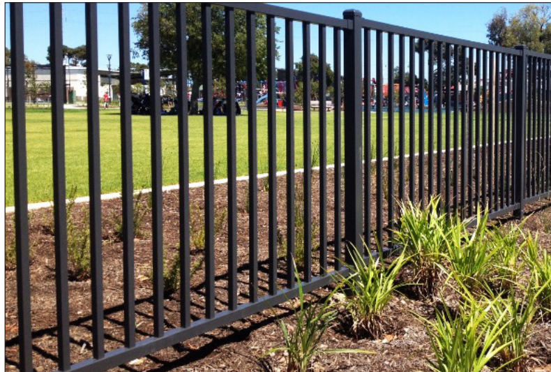
Any future fencing or gates should match the existing fence style that is located along Main Street.
