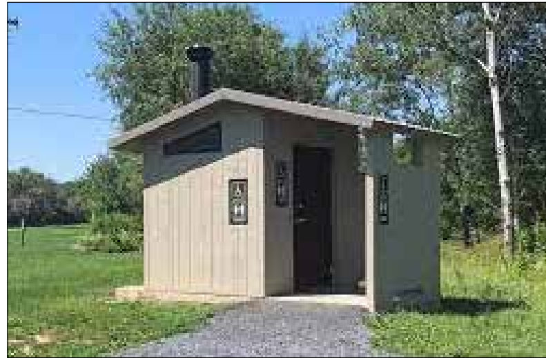
A precast restroom building identical to the one pictured above was recently purchased and will be installed on the site soon.
