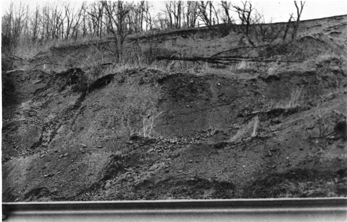
Figure 2—WHAT IF YOUR HOUSE HAD BEEN HERE? This is a landslide in Frederick cherty silt loam. It covers a 360' by 365' area, and thousands of dollars were spent moving it. (See Fig. 3. below)
