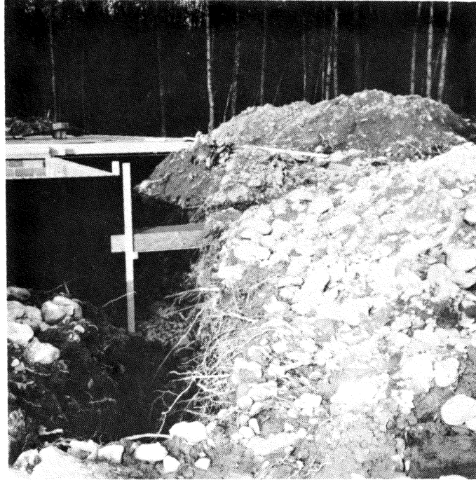
Figure 32—House basement on Holston very cobbly loam. In many places these soils are so cobbly on the surface that good topsoil has to be hauled in to make good lawns.
