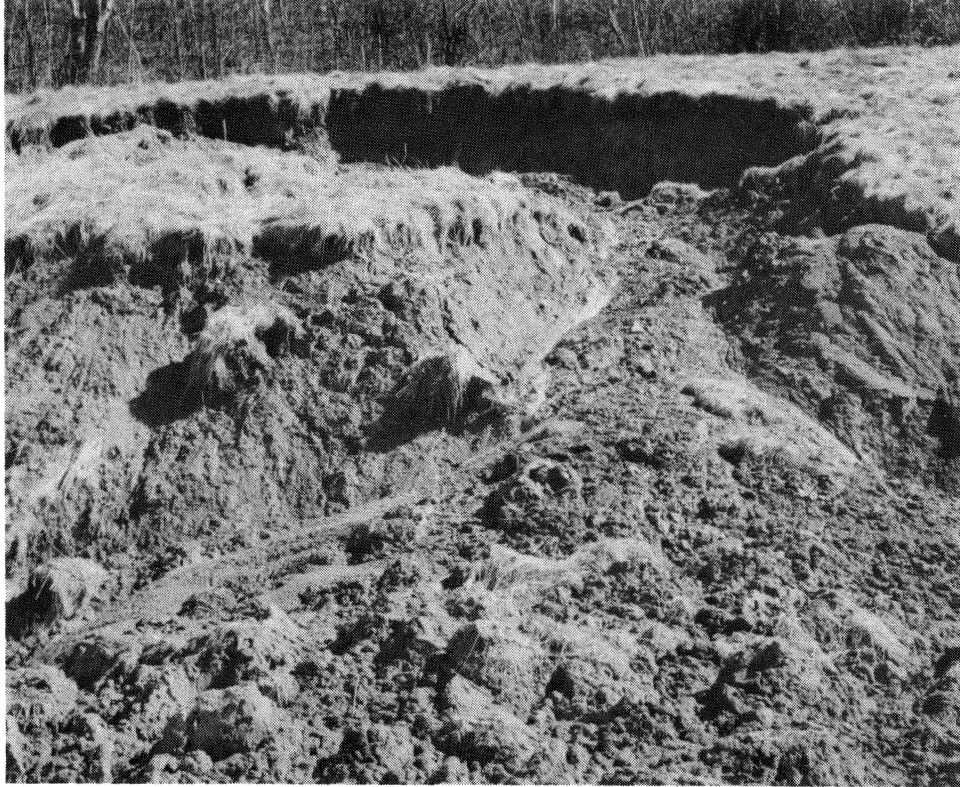
Figure 4—A small landslide in Saltville, Virginia in clayey materials in a fault zone of the McCrady formation. Soil scientists prevented the spending of thousands of dollars by properly evaluating damages which could have resulted from this slide. Proper identification showed that only a small portion of the slope to be loose clay which could slide, where great damage to houses had been anticipated.
