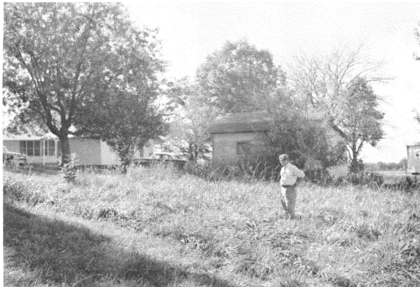
Figure 20—A COMPLETE FAILURE. The tall fescue is growing on a septic tank drainfield that is running over on the surface. This happens frequently in shallow to bedrock shales or in soils that have slowly permeable subsoils. This drainfield was abandoned soon after the picture was taken.
