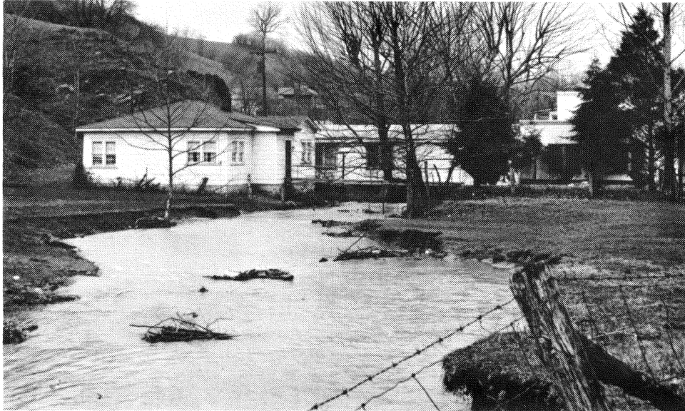
Figure 6—AN UNHEALTHY AND DANGEROUS SITUATION: the owner says this building is damaged by flooding nearly every year, but adjacent soils are too steep, stony and shallow to build on.
