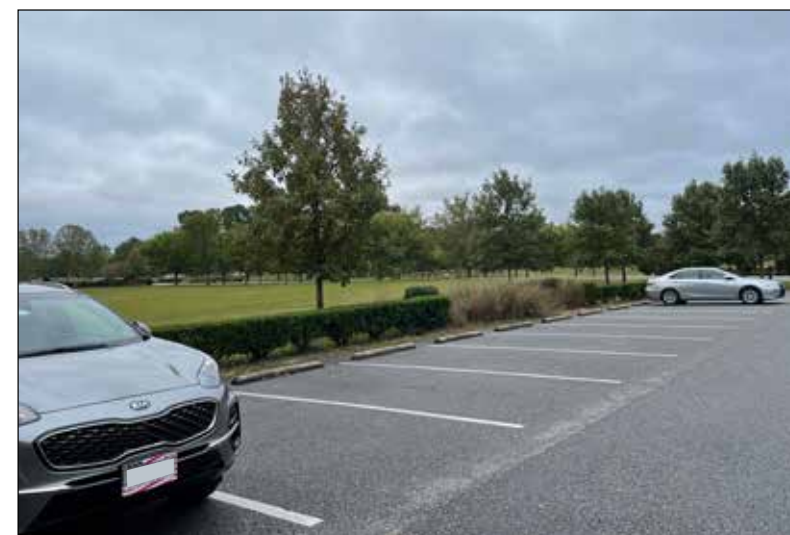
3: Partial view of existing parking lot, which is paved asphalt and has twenty-eight standard parking spaces and one two-way access point.
