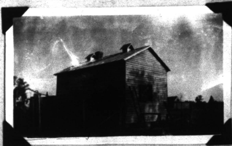
1000 bushel, individual sweet potato storage house. Plan J-8. Virginia has many such houses.
