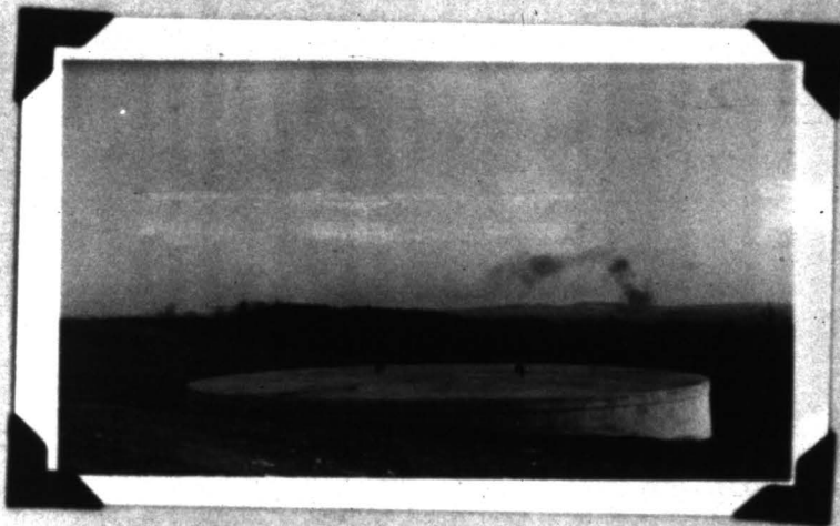
300,000 gallon main reservoir near Country Club House. Blacksburg Water Works
