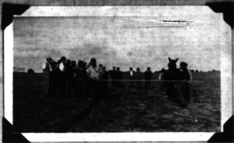
Boys Club Terrace Construction Demonstration Hicklenburg County
