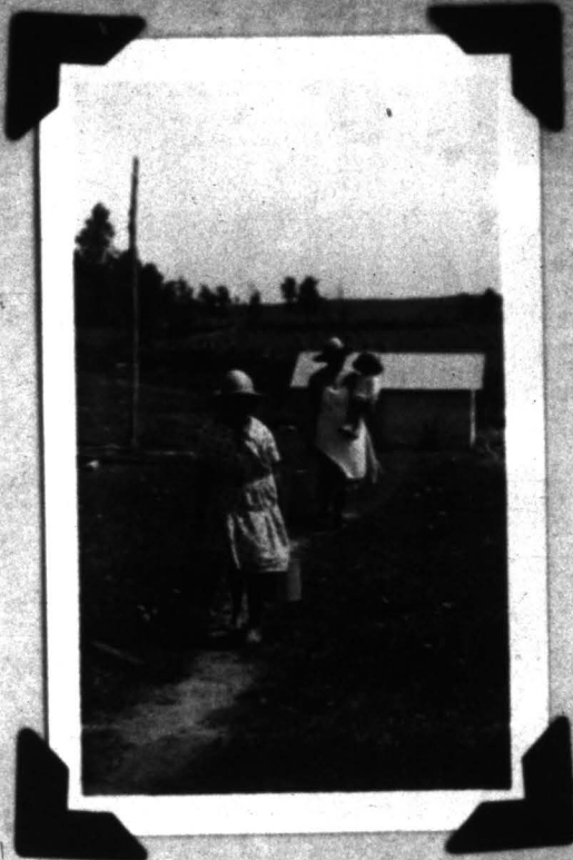
This family obviously needs a water system. A survey has been made and a small hydraulic ram will supply all water requirements.
