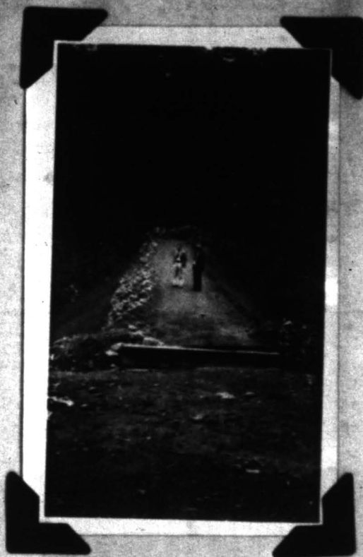
Dam for Fish Pond - Top View Campbell County
