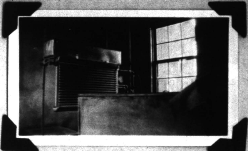
Interior view of dairy house showing cooling equipment
