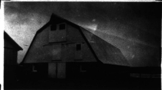
40 cow two-story masonry dairy barn for Washington market. Plan B-2. As result of stan- dardization of plans cost of such structures has been reduced from $250.00 per cow to $85.00 per cow.
