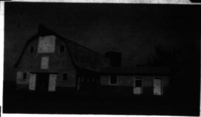
Two-story frame dairy barn and milk house. Prince William Co. Plans B-1, B-24
