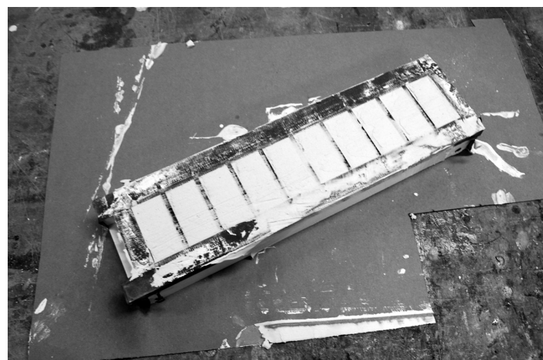
10 plaster units drying in the formwork
