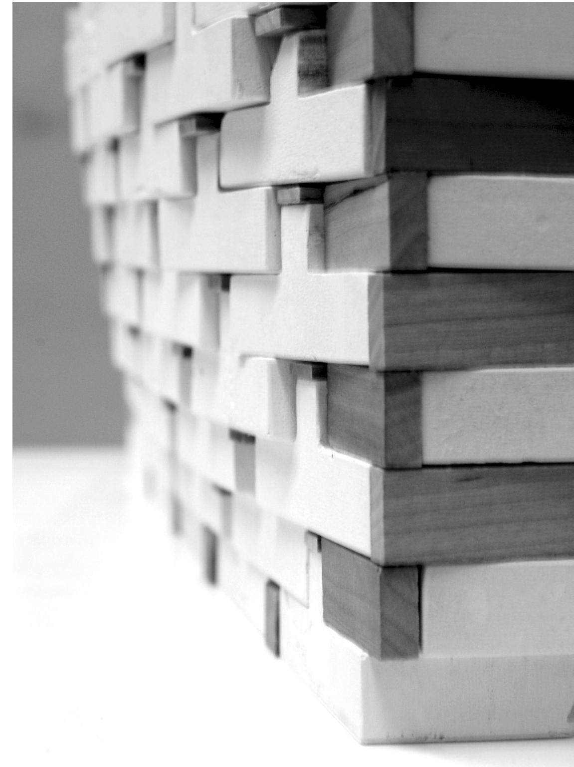
Cut stone is placed in-between the cast T-bricks to express the textile nature of the tower's walls
