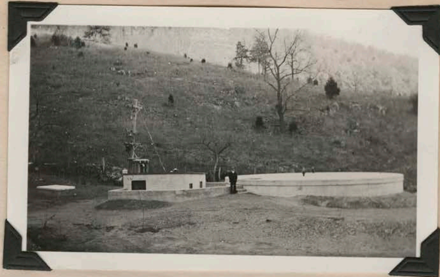
Suction reservoir, transformers, pump house, and treating room. Blacksburg Water Works
