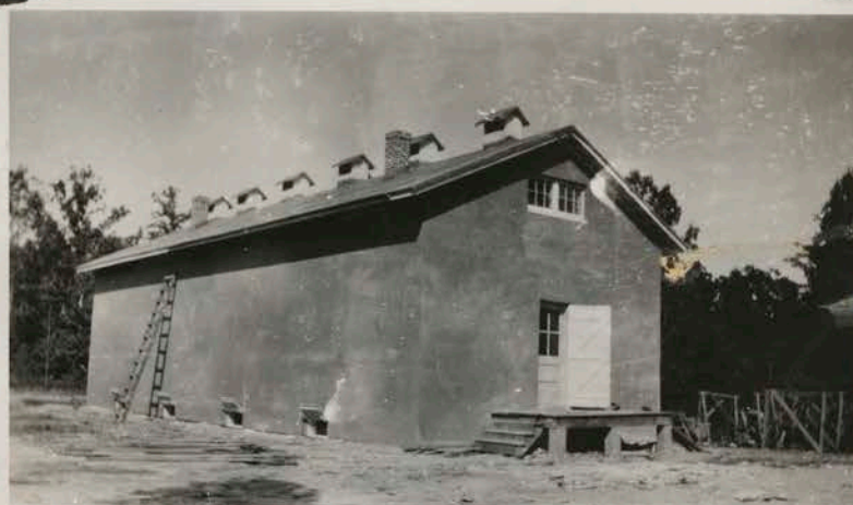
5,000 bushel cooperative cinder block sweet potato storage house Caroline County
