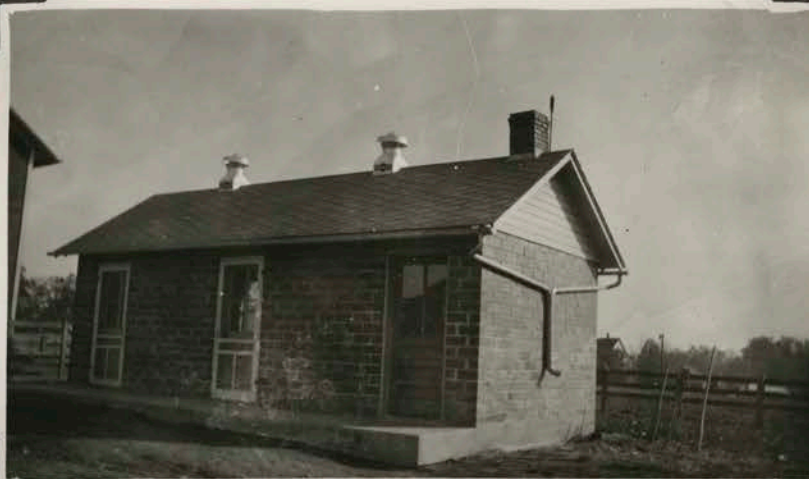
Standard masonry dairy house. Plan B-22
