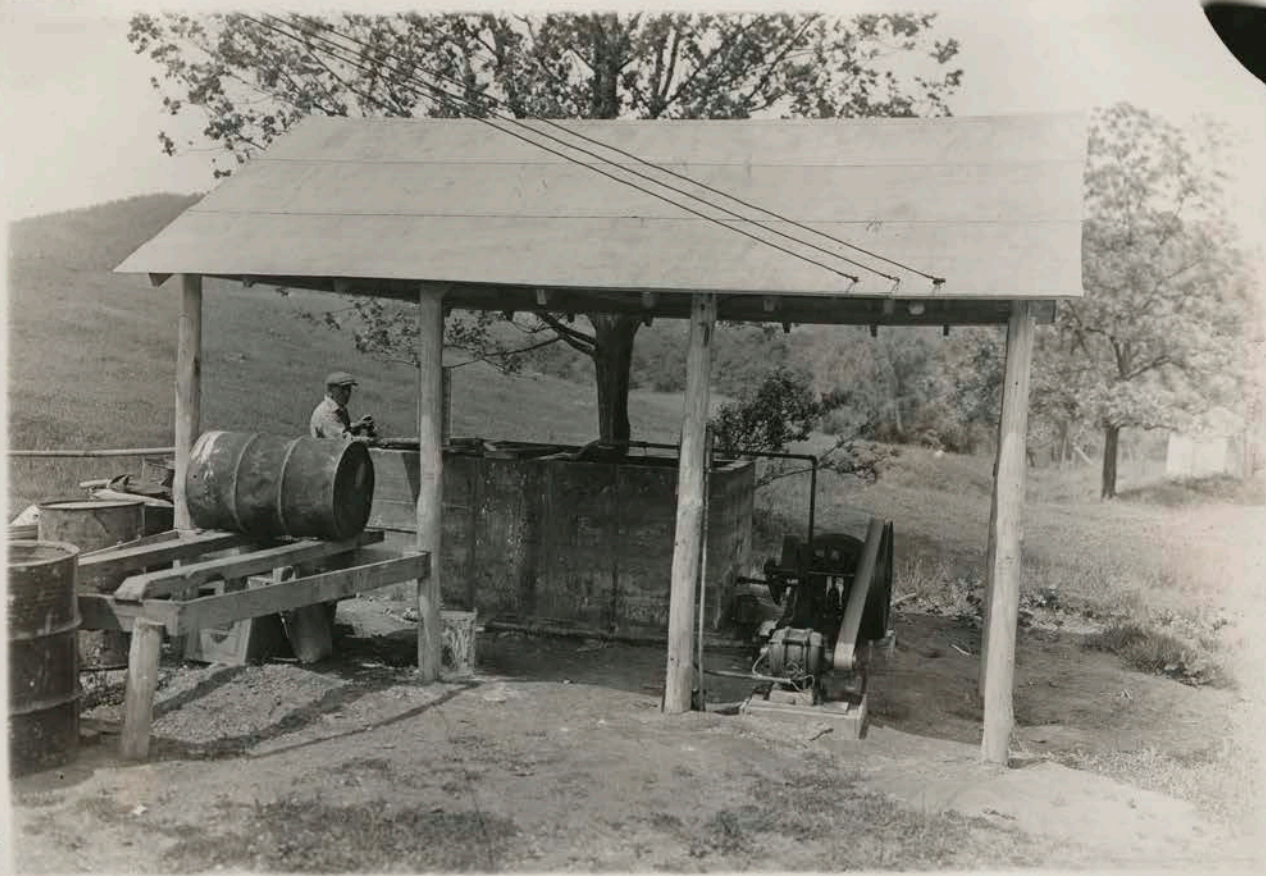
Stationary spray mixing and pumping plant on C. S. Ikenberry orchard. Consists of concrete two-chamber spray mixing tank, high pressure spray pump and electric motor.
