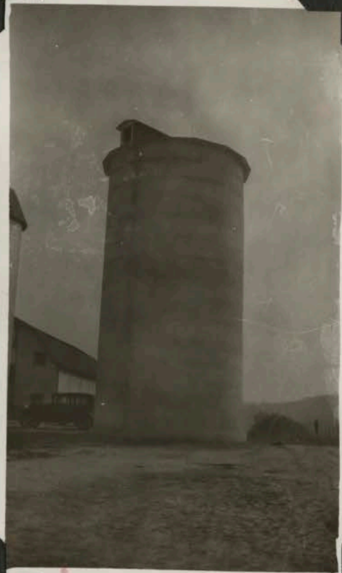
Monolithic concrete silo. These silos are being built for about $2.50 per ton capacity
