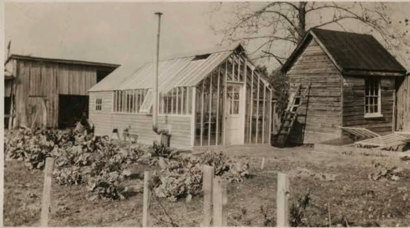
Small sash greenhouse designed for early plant growers. Such houses can be built for $100.00 or less.
