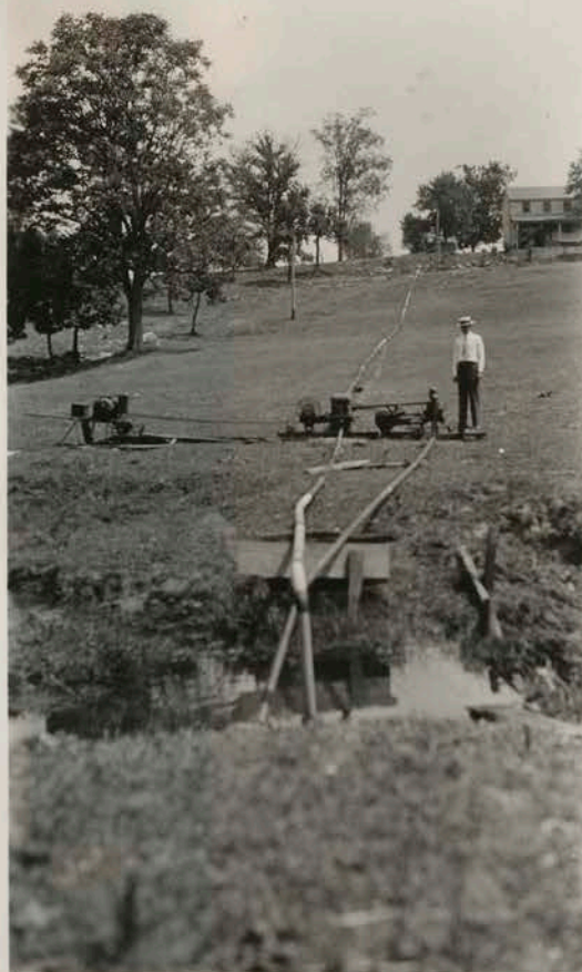
5 H. P. portable farm motor hooked to two pumps on the Bradley farm in Botetourt County. Pumped water for irrigation of 8 acres ensilage corn. This motor also used for cutting ensilage.
