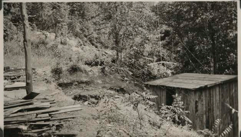
Water power plant of R. Moore, Patrick Co. Turbine, generators, etc., in shed.
