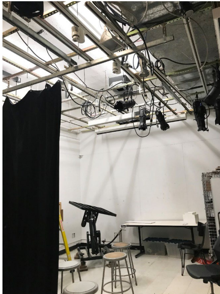
Figure 6-9. Parsons Lighting Lab
