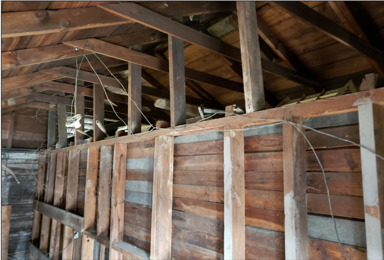
Old wires are seen tacked along the wall and up to the roof.
