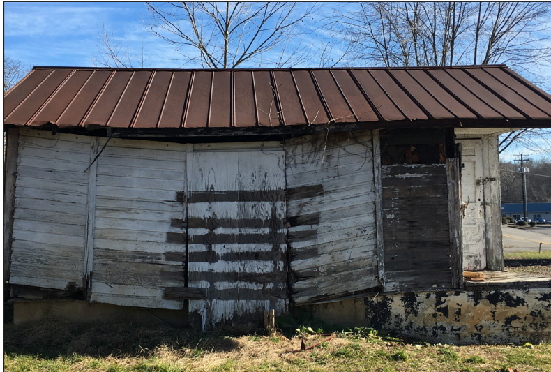
The west facade has the most damage. The exterior siding has begun to sag away from the roof.
