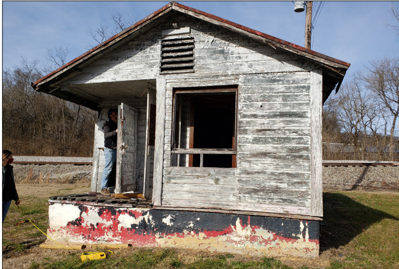
The ice house sits on a 2' concrete slab. This building's construction is thought to be similar to Sears & Roebuck Company's "Simplex" prefabricated type construction.
