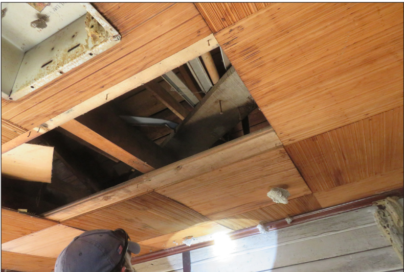
The wood paneled ceiling shows damage and pieces are starting to fall off.
