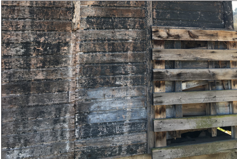
Part of the north side facade of the building is damaged and was repaired with a wood pallet.
