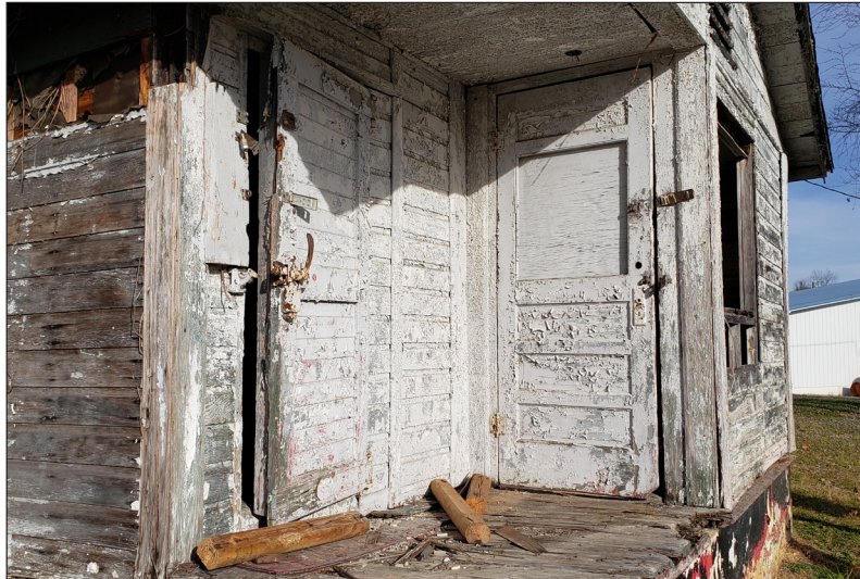
The south facade faces Riverside Drive. The front side of the building includes a small deck with two doors to access the interior. The deck does not have steps and is not easily accessible.
