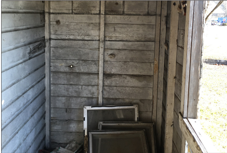
The front room attached to the deck shows paneling similar to the exterior, suggesting this may have been an addition to the original structure.
