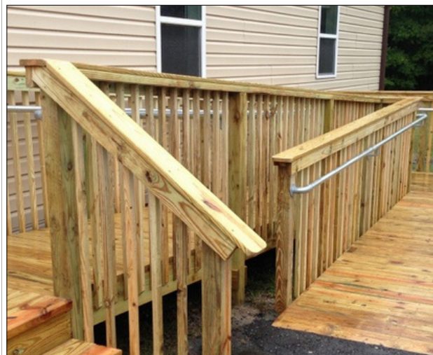
A wood ramp serves as both the main patron entrance and the ADA accessible entrance.
