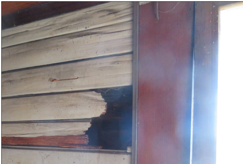
The paneling on the wall shows damage.
