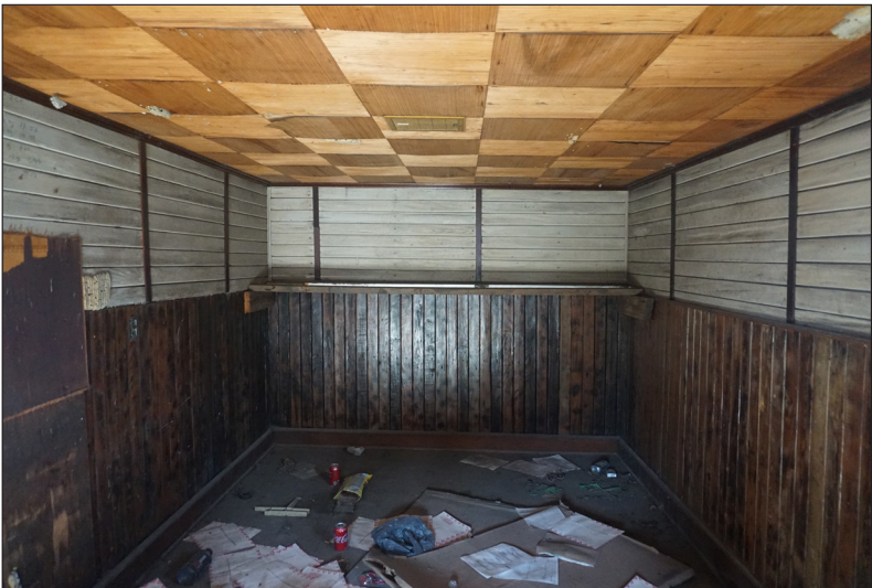
This interior room is located on the east side of the building. The walls and ceiling have wood paneling and the floor is vinyl tile.
