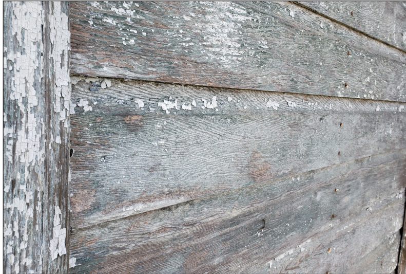
Horizontal wood siding covers the entire exterior of the building.
