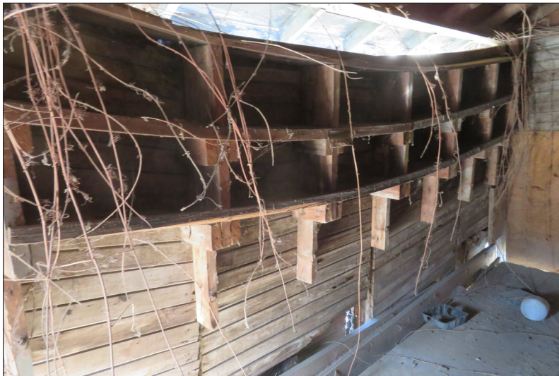
The damage to the west facade is visible from the interior. This image shows the panels sagging away from the roof.
