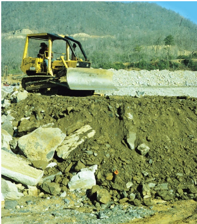
Figure 6. Final reclamation grading of a topsoil substitute. The designated material has been end-dumped in closely spaced piles and is being graded with a small bulldozer. By following the set of practices outlined in this chapter and excluding traffic after final grading, 3 to 4 feet of loose, uncompacted minesoil material can be created in most surface mining environments.
