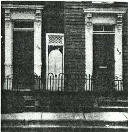
MAIN ENTRANCE - an invitation to a building.
