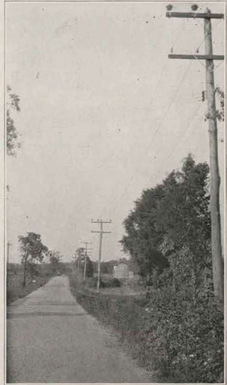
High tension and service line.
