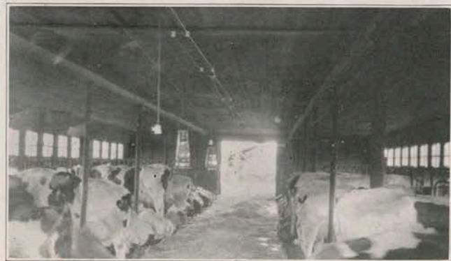
Electric lights replacing lanterns
