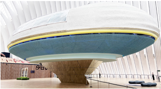
Figure 1: Architectural application of the spatial 3D printing technique: 3D printed lattice designed by Virginia Tech and manufactured by Nagami Design
