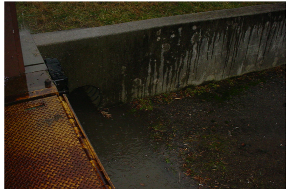
Poor drainage at the loading dock of the existing Kessler Mill building.
