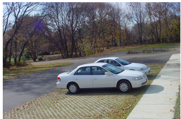
Pavers are used for the parking spaces in this lot while the driving areas are regular pavement.
