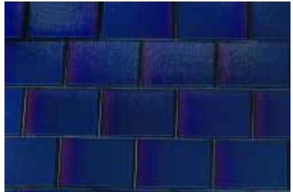
Photovoltaic cells have been used to create roofing shingles. ( www.oksolar.com/images/solar_panels_unisolar_shr17_b.jpg )
