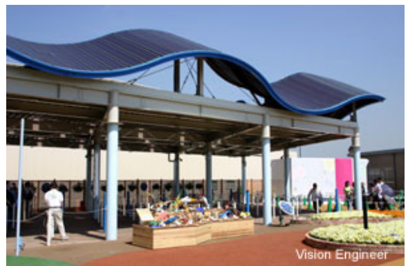
Photovoltaics do not limit the architectural features of a building. (www.visionengineer.com/expo/curved_photovoltics.jpg)
