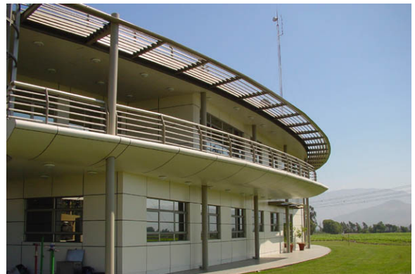
An example of louvers on a building blocking the sun. ( www.hunterdouglas.cl/english/products/sun/photos/zoom/Aero01.jpg )
