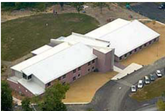
A white EnergyStar roof lowers the temperature of the roof by reflecting the sun. ( /www.hersheyphilbin.com/news/css/images/londonderry.jpg )
