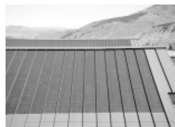
Figure 8: Example of standing seam roof
