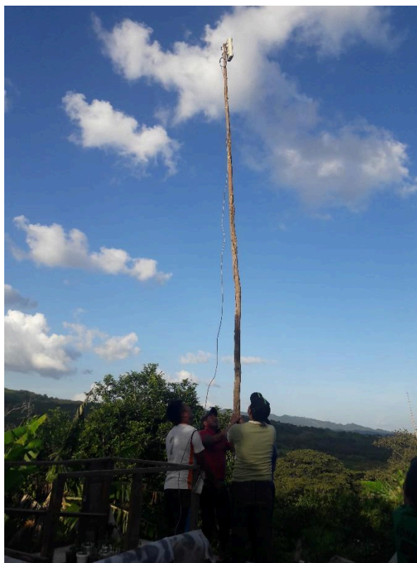
Figure 2. Placing an Antenna in Abasolo, Ocosingo, Chiapas 10
