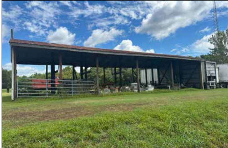
L1: View of livestock building looking east towards western side of the building.
