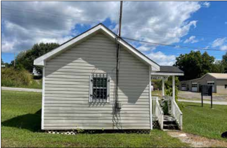
O5: View facing east toward west facade of building.
