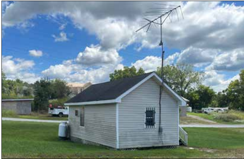
O6: View facing southeast toward north and west sides of the office. This image also shows the satellite antenna on top of the building.
