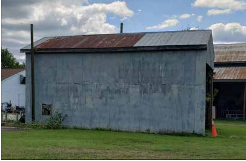
S2: View of building looking west. The BDX performance building and vacant southern states building are located in the background.
