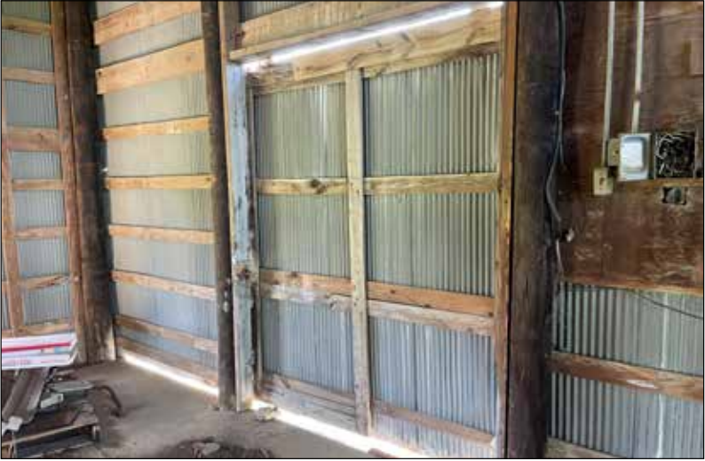
S6: View of barn door located along west facade.
