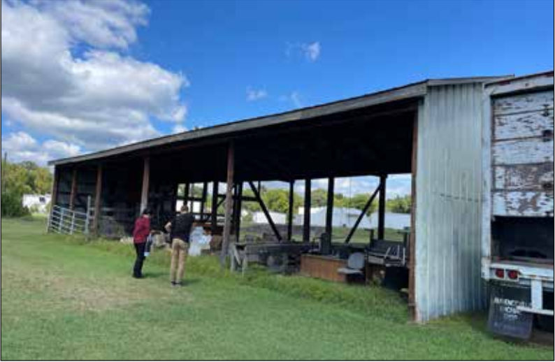
L3: View of livestock building looking northeast toward western side of the building.
