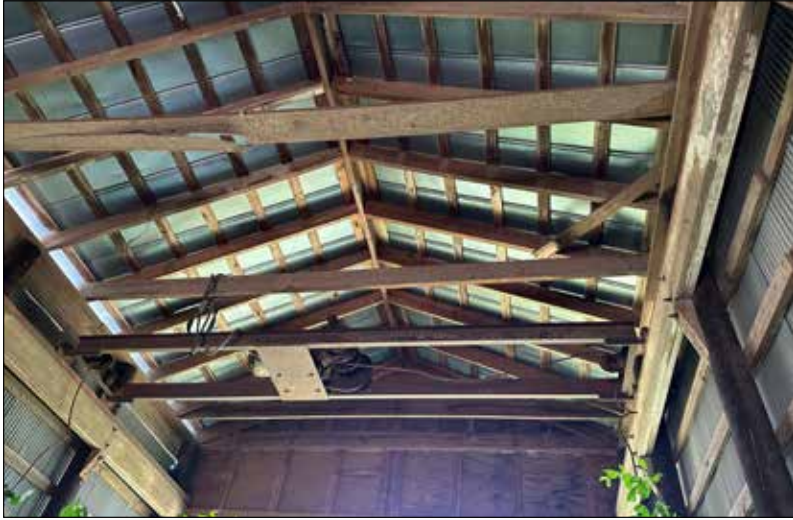
S5: View of interior ceiling. It appears a garage door was once used to control access to the north facade.
