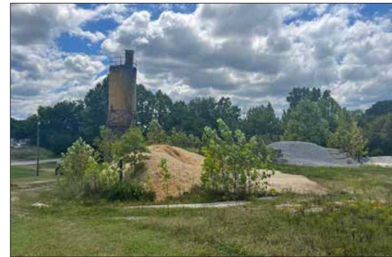
11: View looking south showing part of the materials yard for Felton Bros. Transit Mix and the tower. Materials could potentially be relocated or reused onsite.
