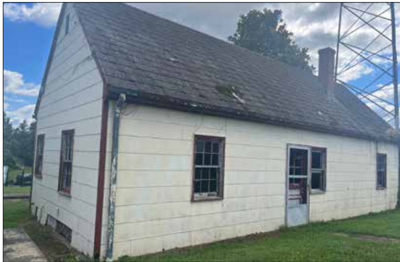
S1: View of the scale building exterior facing southwest.
