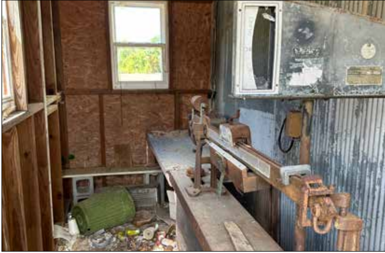
S8: View inside the building's storage attachment.
