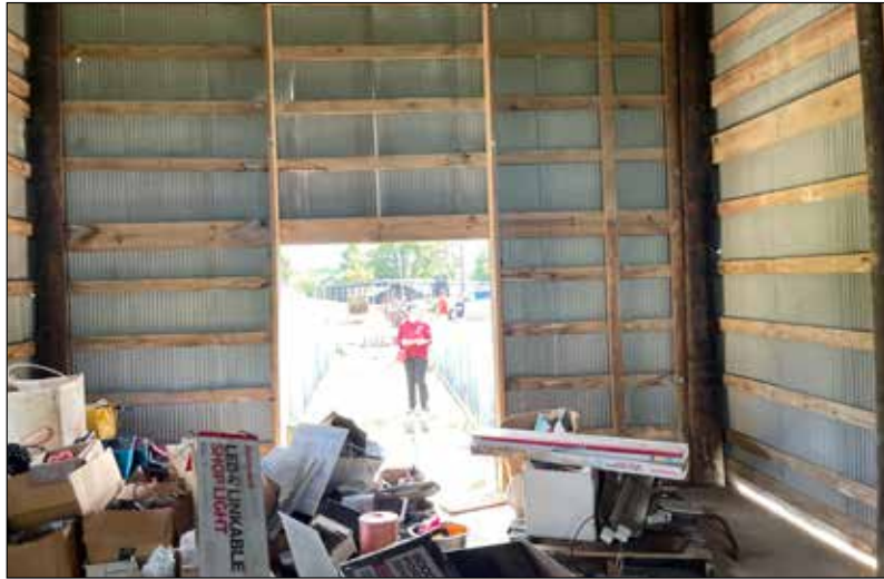
S7: Interior view looking south.
