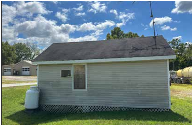
O7: View facing south toward north facade of building.
