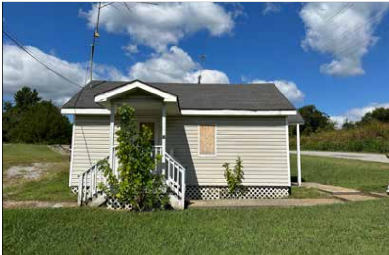
O3: View facing north toward south facade of the building.
