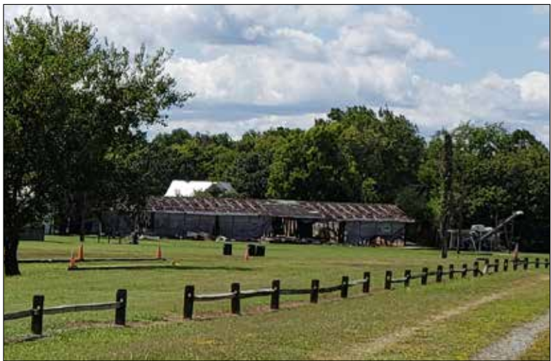
1: This image looking west shows part of the Tobacco Heritage Trail, remaining rail infrastructure, and the former rail car repair shed.
