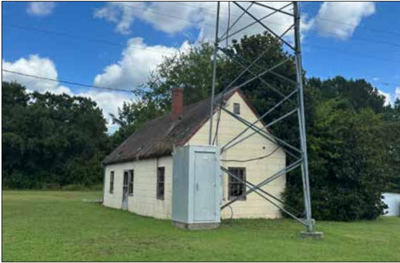
S2: View of the building exterior looking east. The fire department repeater is located next to the building.
