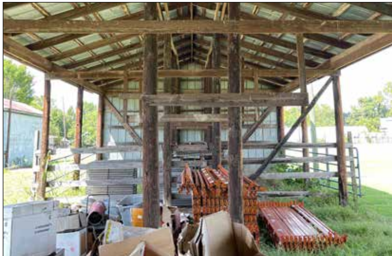
L7: While the structure lacks walls, its wood support beams appear to be in good condition.
