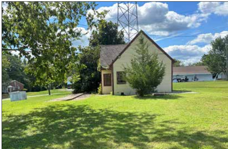
S4: View of the building exterior facing east. Rail tracks still remain just south of this building, though their exact purpose or function is unknown.
