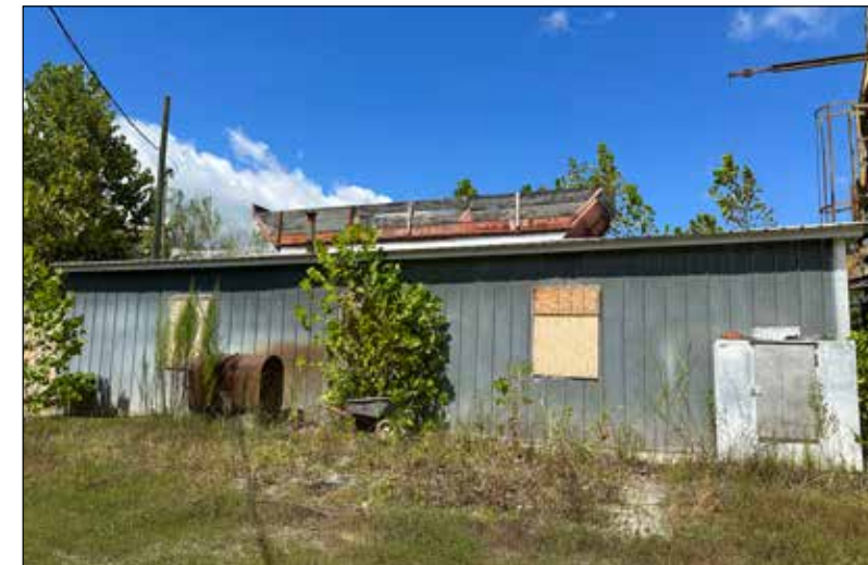
12: View looking north towards the concrete plant structure, which is built into the side of a slope and appears to have some sort of machinery attached to the roof.
