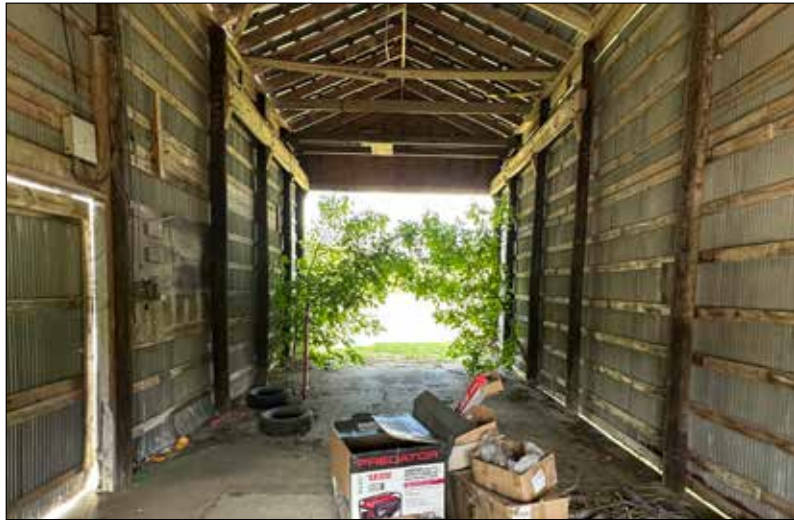
S4: The north face of the building is currently open.
