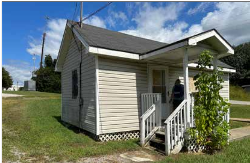
O4: View facing northeast toward the south and west facades of the building.
