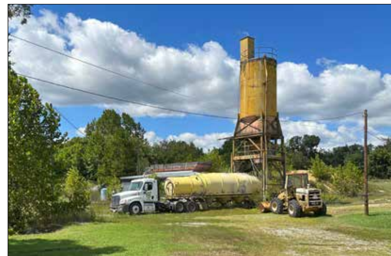
13: The concrete silo is located behind the Felton Bros. Transit Mix office and will be removed during park development.
