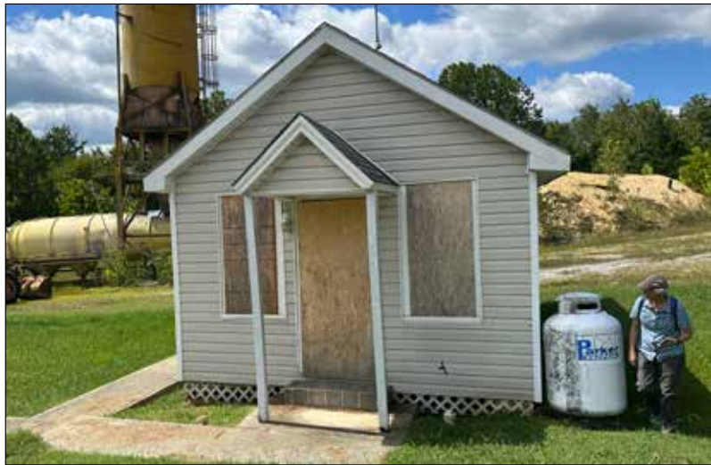
O1: View facing west of east facade of building with the concrete tower in the background.
