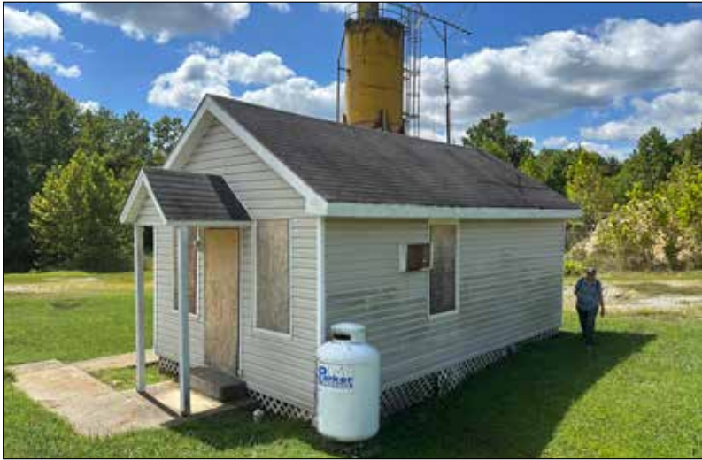
O8: View facing southwest towards northeast facade of building.
