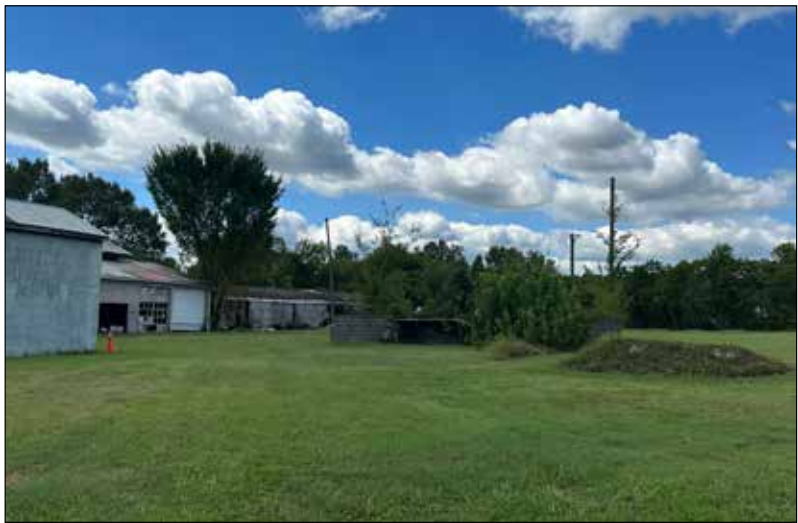
2: This image captures the northern end of the maintenance garage, the vacant former Southern States building, the former rail car repair shed, and remnants of an additional building foundation.
