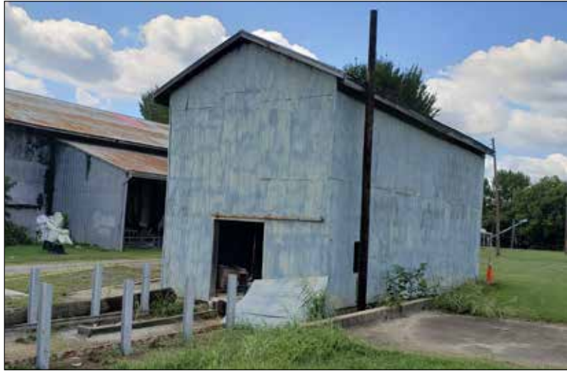
S1: View of building looking northwest.
