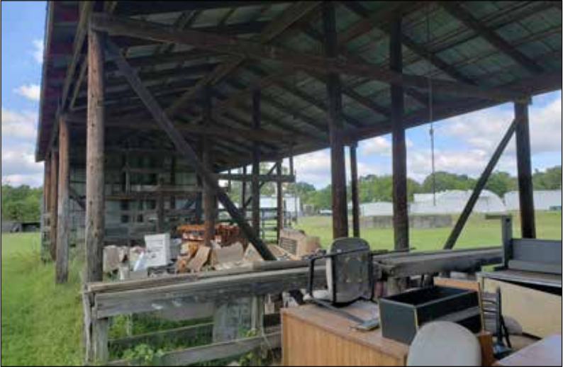
L6: An additional interior view of the building looking north towards the livestock pen.
