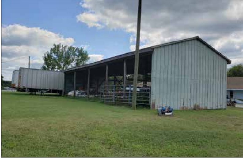
L2: View of livestock building looking southwest towards east facade of the building.
