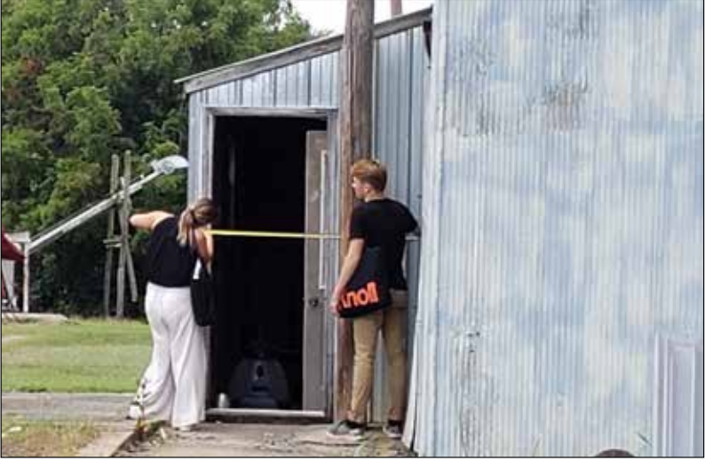
S3: View of the storage attachment, which is located along the building's west facade.
