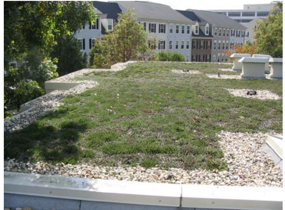
Green Roof, Yorktowne Square Condominiums, Falls Church, Virginia
