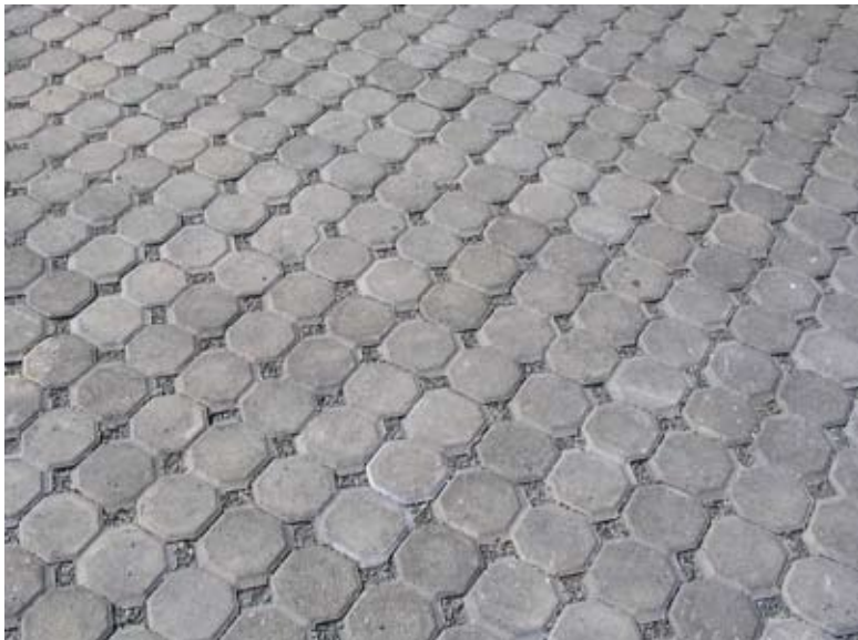
Permeable concrete pavers
