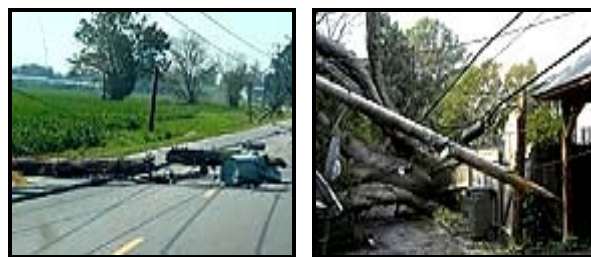
Power-system damage. Photos from Dominion Virginia Power; used with permission.
