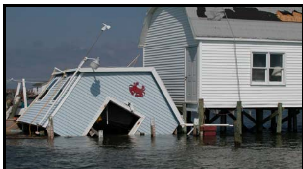
Storm damage on Tangier Island, Va. Photo by George Roarty, Va. Dept. Emergency Management.
