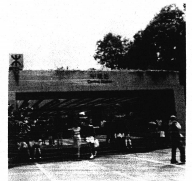
Figure 19. Mass Transit Railway Station
