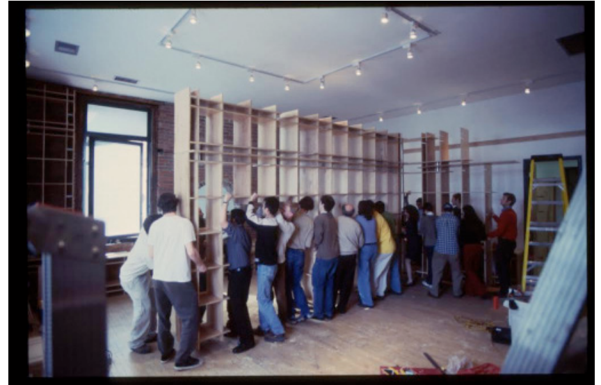
Students and faculty setting up the design-build bookshelves at the library Photo Credit: WAAC Archives
