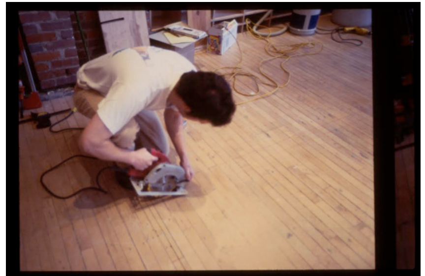
Student placing the flooring of the library Photo Credit: WAAC Archives
