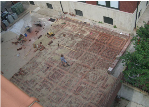
Student and faculty working on laying the brick courtyard ( http://arch-design.vt.edu/programs/waac )
