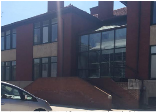
Back Terrace- the finished floor elevation (F.F.E.) of the terrace at 4 feet higher than the parking level Photo by (Elyana Javaheri)
