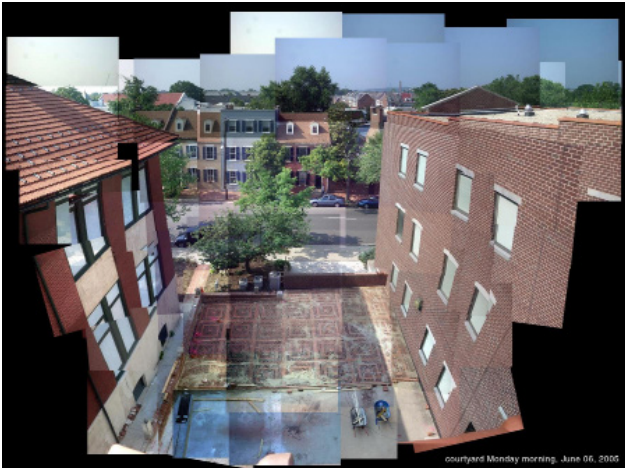
Courtyard in process of being built Photo Credit: WAAC Archives
