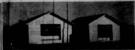
Two crop drying bins, each 20'x30' on the farm of Millard Turner, Broadway, Virginia. The portable crop drier is located between the bins. The drier is connected to a main duct between the bins and air can be forced into either one. Each bin has a perforated metal floor for drying small grain, corn or baked hay.
