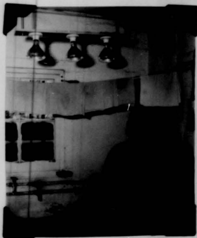
Infrared lamps can be used for many other purposes besides brooding. This Franklin county dairy farmer installed three infrared lamps over the wash vat in the milk room to provide warmth for washing utensils. Several farmers in Virginia are using this source of heat in their milk rooms.
