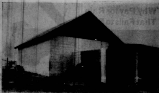
Hay drier on J. E. Hawkins farm, Chesterfield County, Virginia. Drying building is 20 ft. by 30 ft. Note open gable for escape of moist air. Crop-drier is located in air tunnel at right of picture. Fuel oil tank is beside air tunnel.
