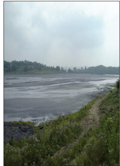
FIGURE 4.20 Active slurry impoundment used for fine waste disposal (before reclamation).
