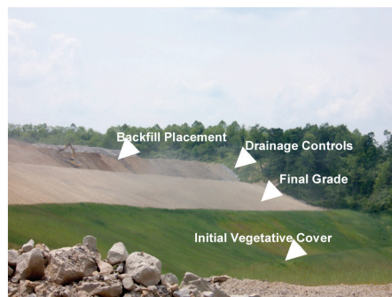
Backfilling in Progress in Mountaintop Mining
