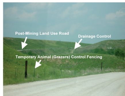
Backfilled Area, Graded to AOC (Prior to Reforestation)
