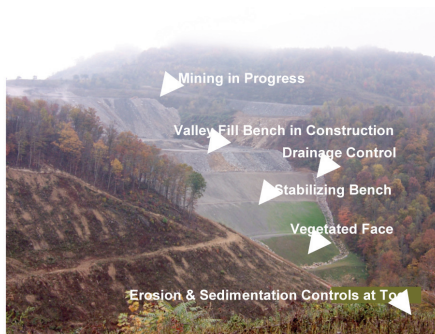
Valley Fill (Excess Spoil Storage) Under Construction
