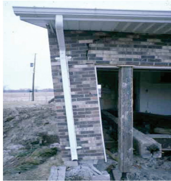
FIGURE 6.9 Impact due to land subsidence. Freeburg, IL. SOURCE: Illinois Department of Natural Resources, 2008. http://dnr.state.il.us/mines/aml/gallery/freeburgc.html .
