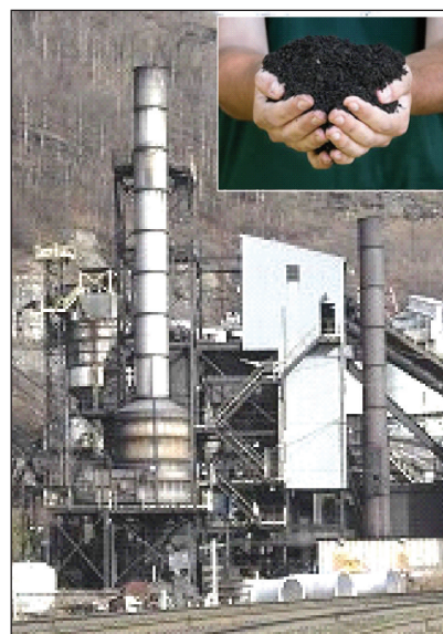
FIGURE 4.18 Thermal dryer used to dry coal to low moisture contents.
