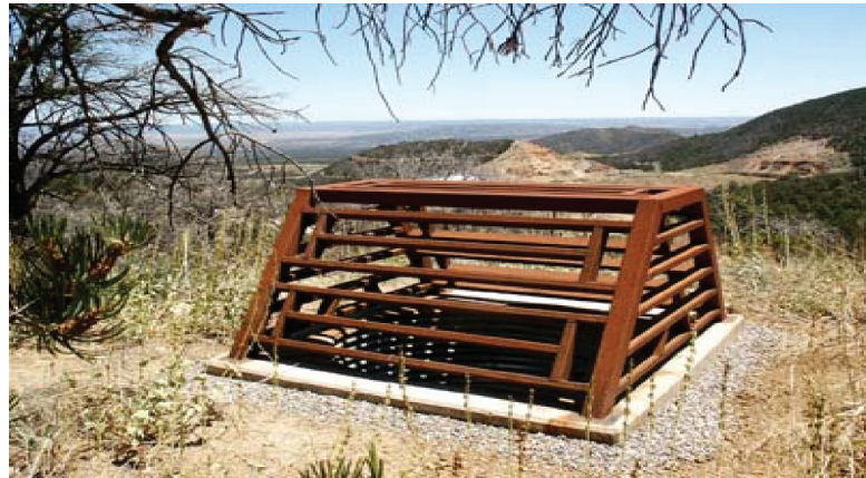
FIGURE 6.13 English bat cupola at an abandoned mine. SOURCE: OSM, 2007a.
