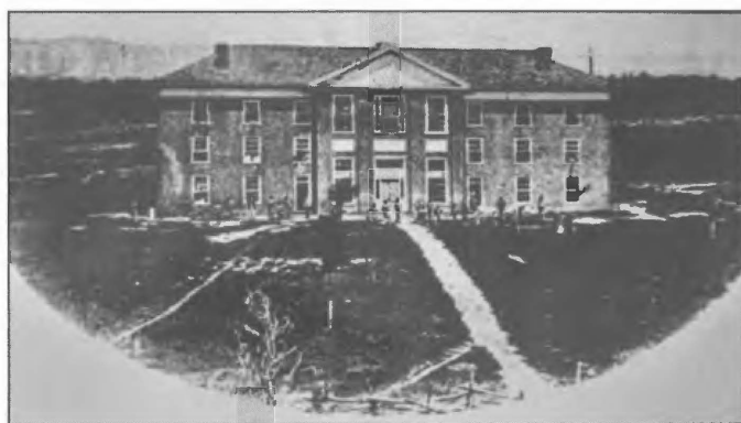
Figure 6. This three-story brick building, completed in 1855, was the subject of a long-running lawsuit filed against Olin and Preston Institute by the contractors who built it and remained unpaid. Courtesy Special Collections, University Libraries, Virginia Tech, Blacksburg, Va.
