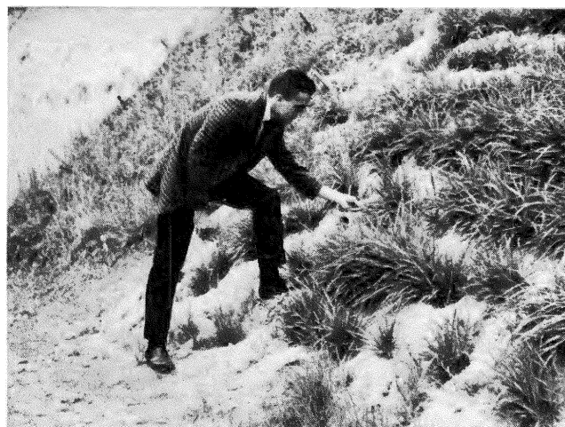
Lateral furrows cut on steep roadbanks improve sod establishment. Plot at upper left in picture did not have furrows.
