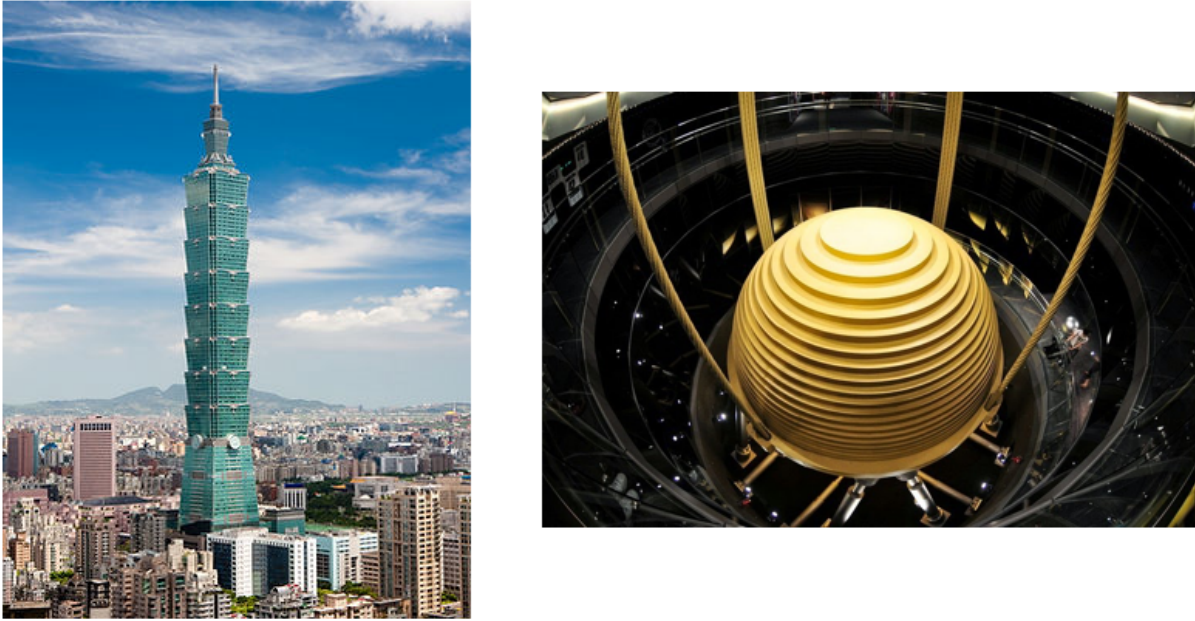
Figure 2.11: Image of Taipei 101 in Taiwan and of the pendulum type TMD located within the tower
