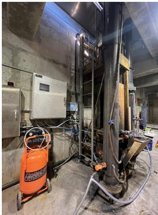
Figure 65: Pilot feed flow setups - the final waste and feed iteration with 2-inch and 1-inch, respectively, batched daily powered by air actuated ball valves.
