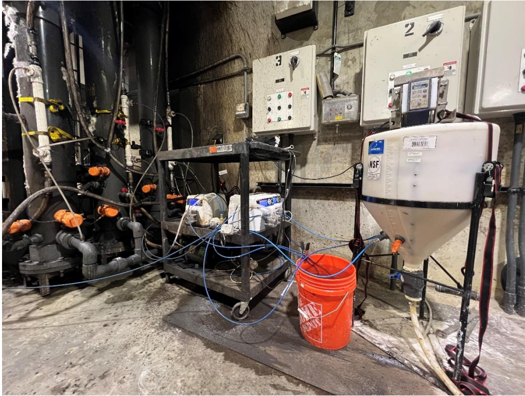
Figure 5: Chemical dosing setup for the pilot.
